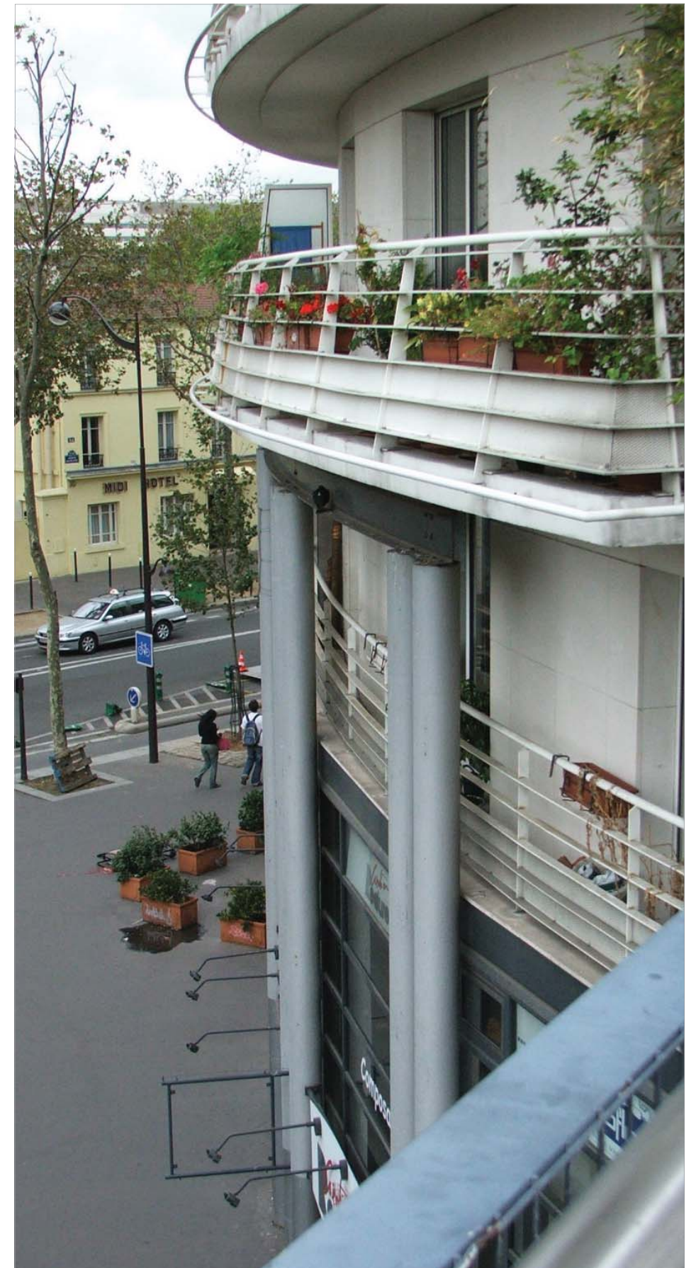
Rounded corner of residential building with balcony
