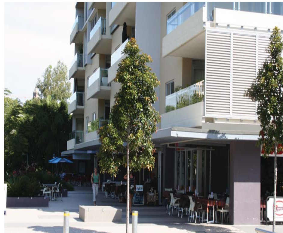
Consistent and continuous awning frames pedestrian area
