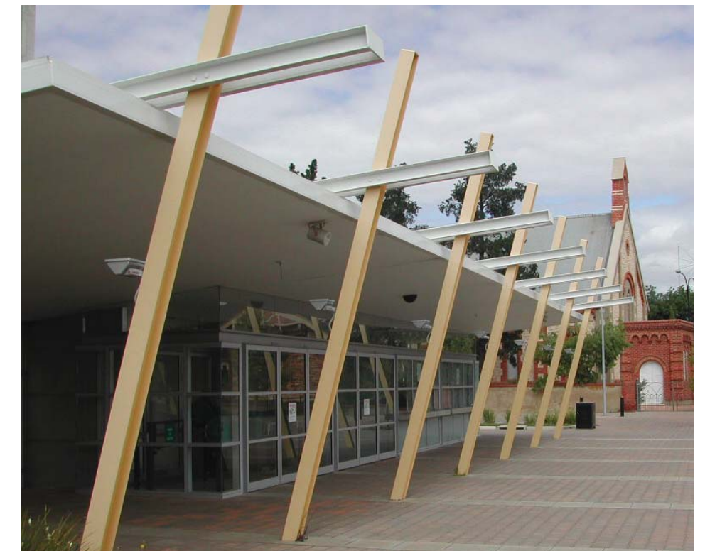
Metal awning posts echo line and colour of heritage church
