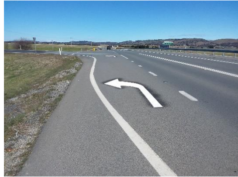
Photo 31: Kings Highway and Old Trucking Yard Lane intersection
