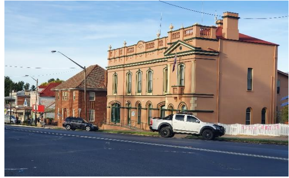
Photo 26: Braidwood office building
