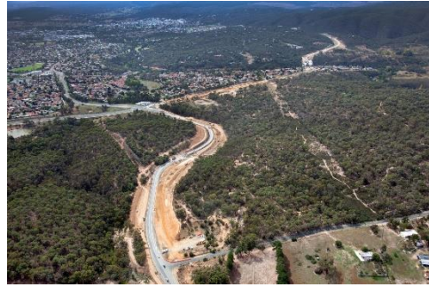
Photo 27: Road Construction: Old Cooma Road and Ellerton Drive Extension
