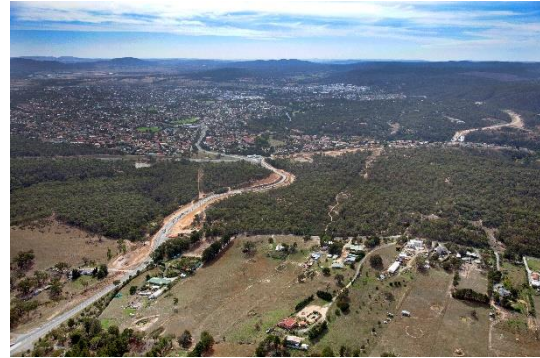
Photo 20: Old Cooma Road realignment for Googong
