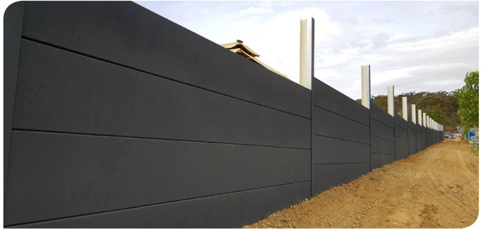
Image of partially completed noise wall along Ellerton Drive, transparent panel to be installed above concrete panels.
