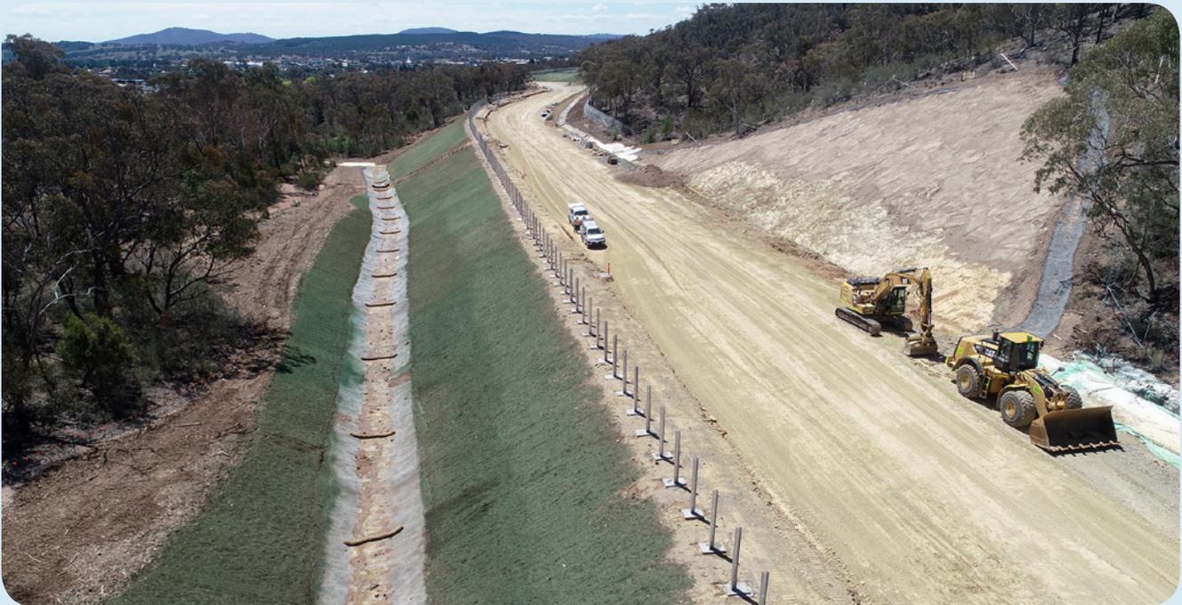
Image of revegetation work and steel posts installed for noise wall construction
