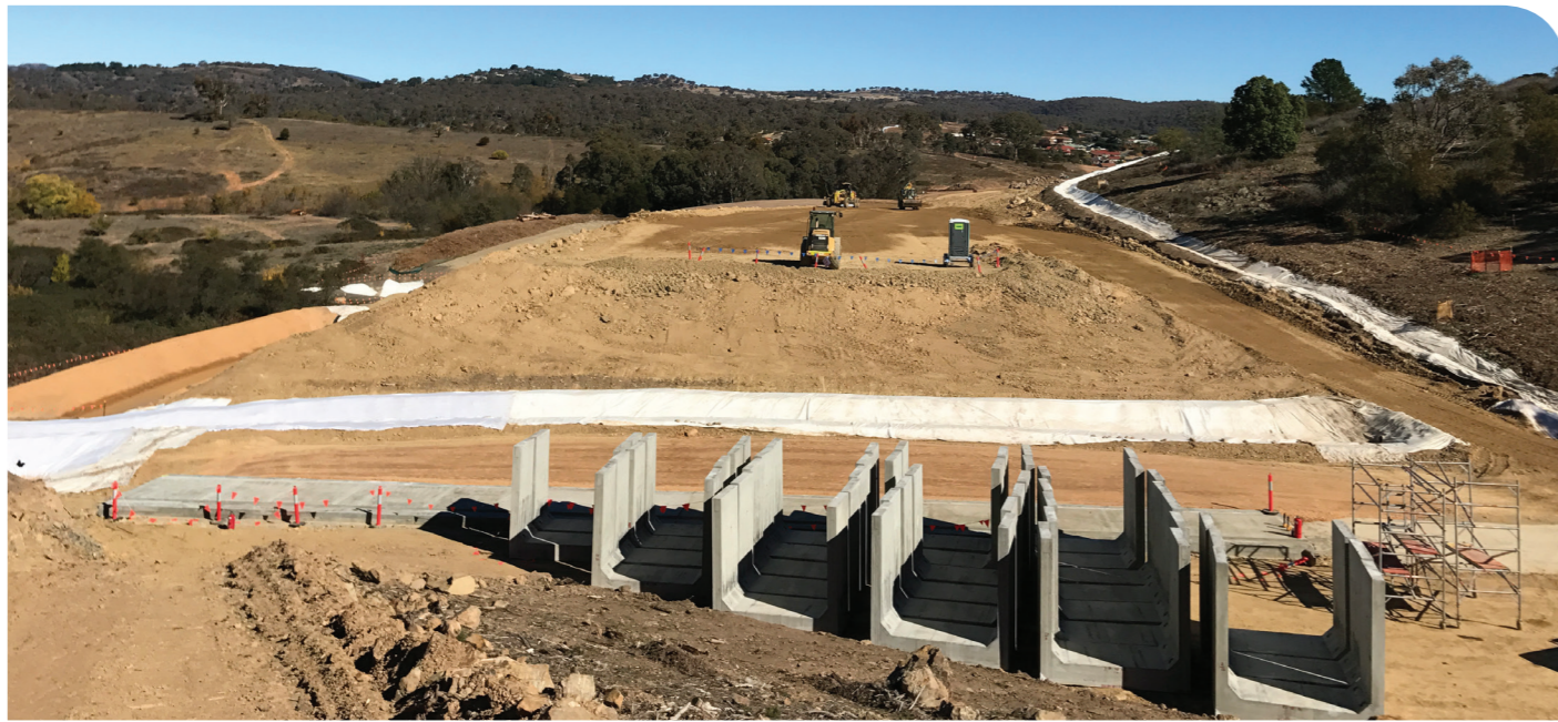
Fauna underpass construction and earthworks at Greenleigh
