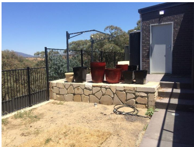
Figure 5: New 700mm retaining wall return
