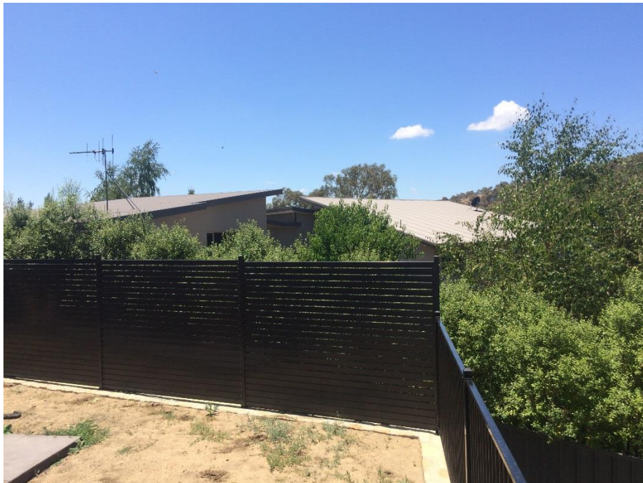
Figure 2: Installed 1.8m powder coated steel privacy screen
