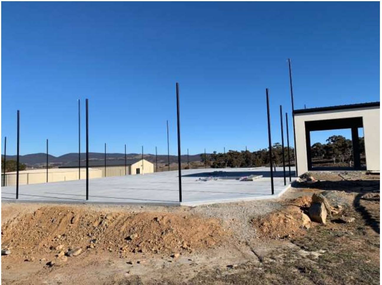
Figure 2 Site of proposed development showing completed works.
