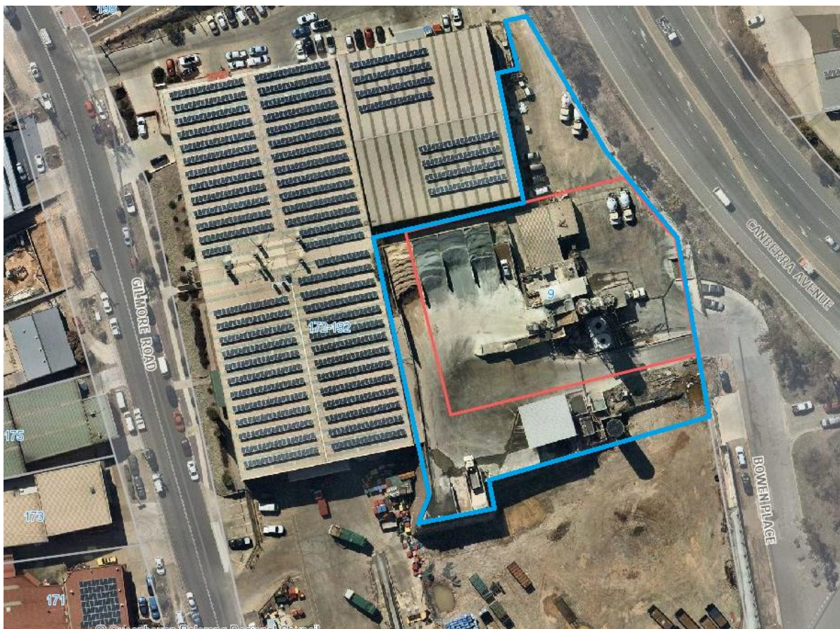
Figure 2 – Extent of Concrete Batching Plant
