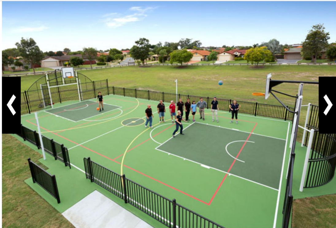
Figure 5: Example of multi-sports court, recently installed by the Brisbane City Council
