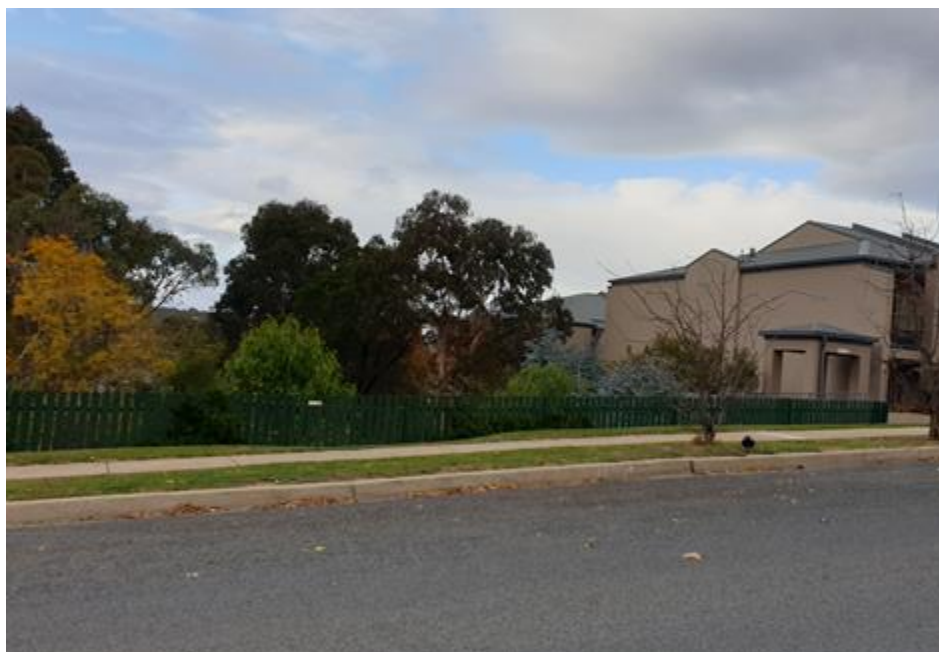
Figure 2: Subject site as viewed from Antill Street
