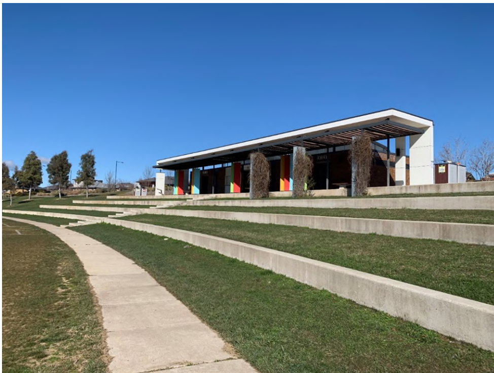
Figure 3 Rockley Oval facilities
