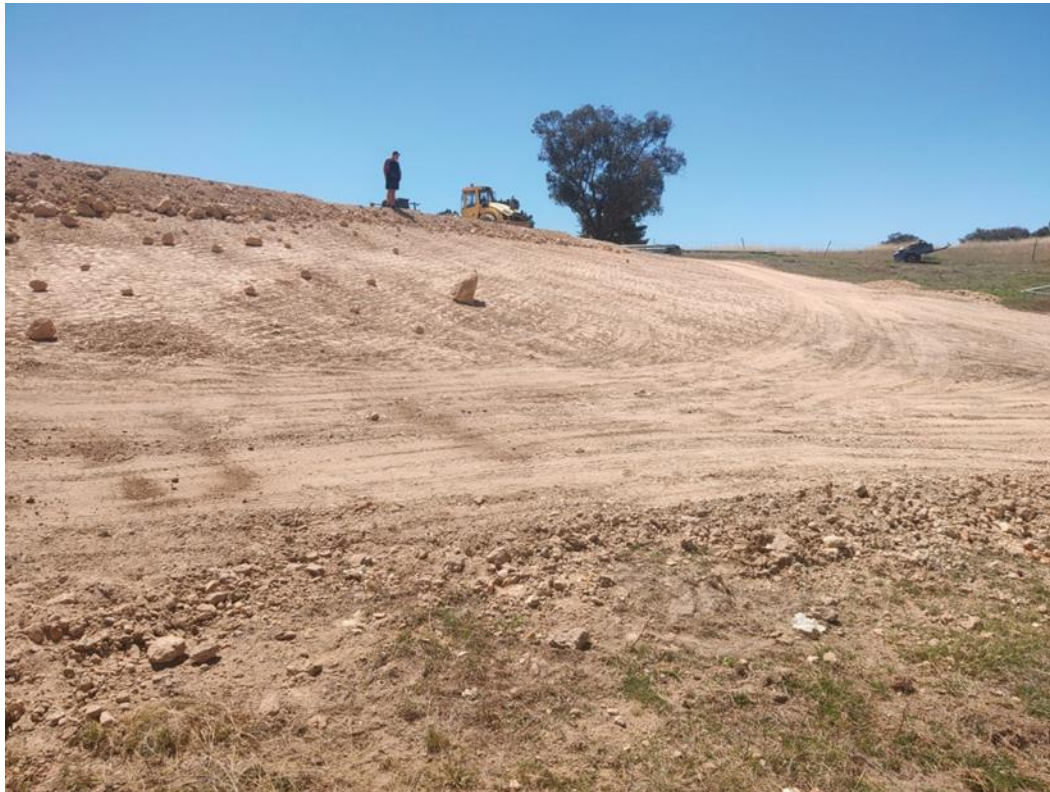
Figure 8: Fill Used to Level the Proposed Siting of The Farm Building
