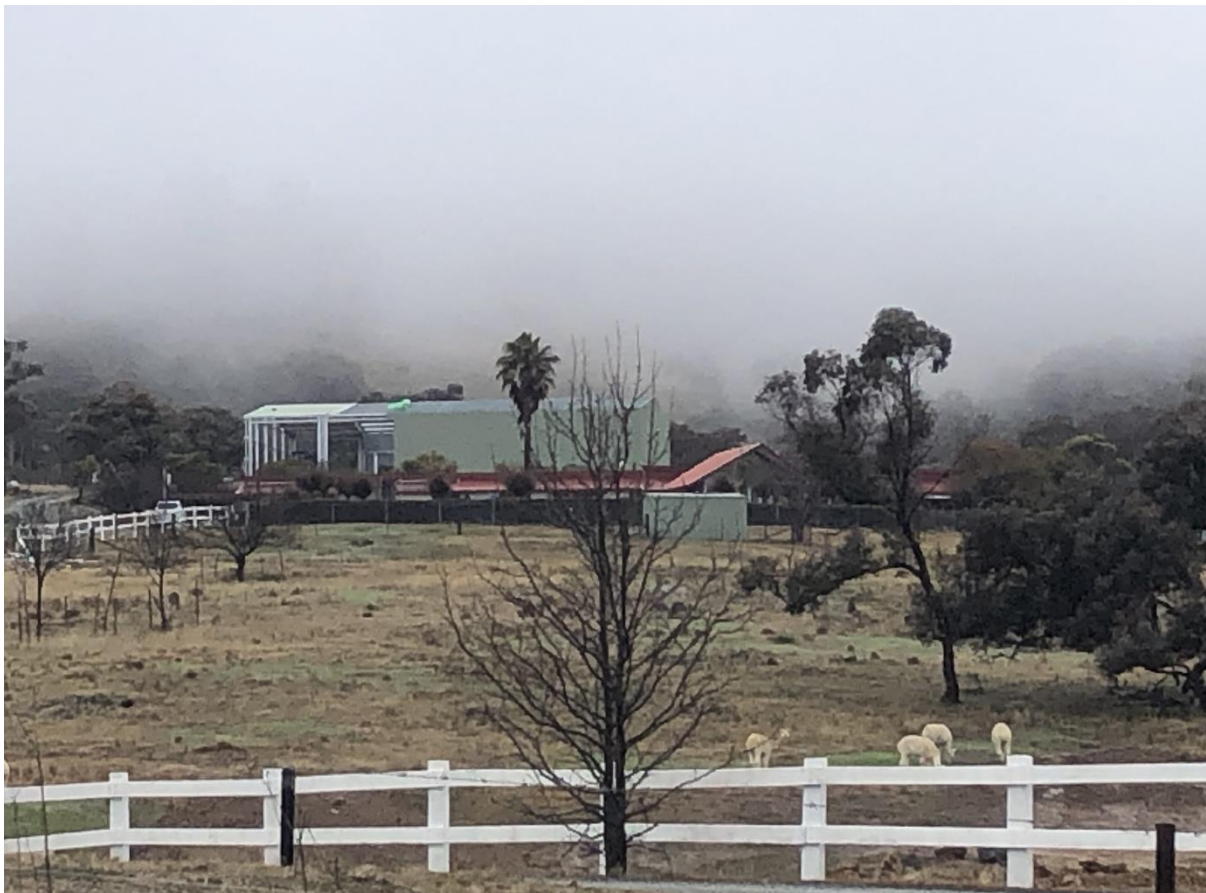
Figure 9 – View of Partially Completed Shed from Fernleigh Drive – 21 July 2021.
