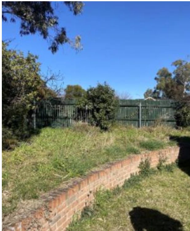
Figure 11 – Photo of existing retaining wall (Gold Leaf Arborist Report)
