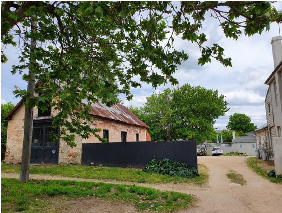
Figure 7 – Brick Stables (retain) from Duncan Street
