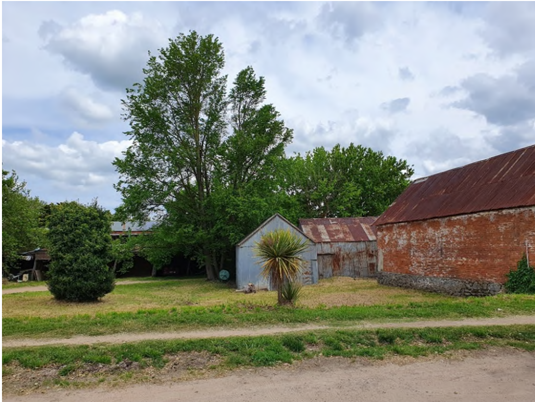
Figure 5 – T-Shaped Shed (demolish) and Brick Stables (retain) from Duncan Street
