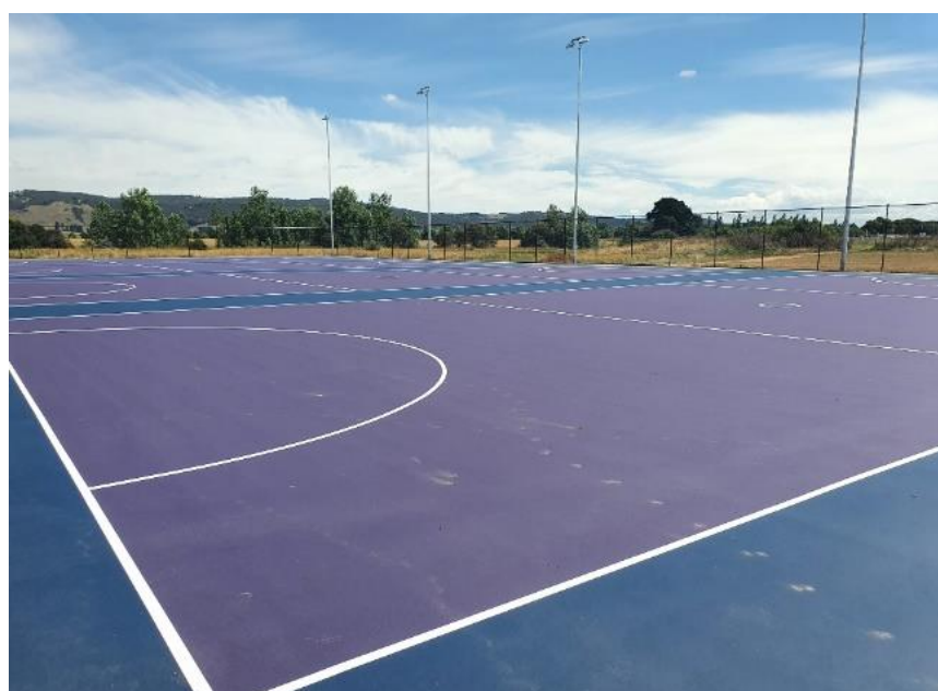
Figure 2 – Completed Netball Courts
