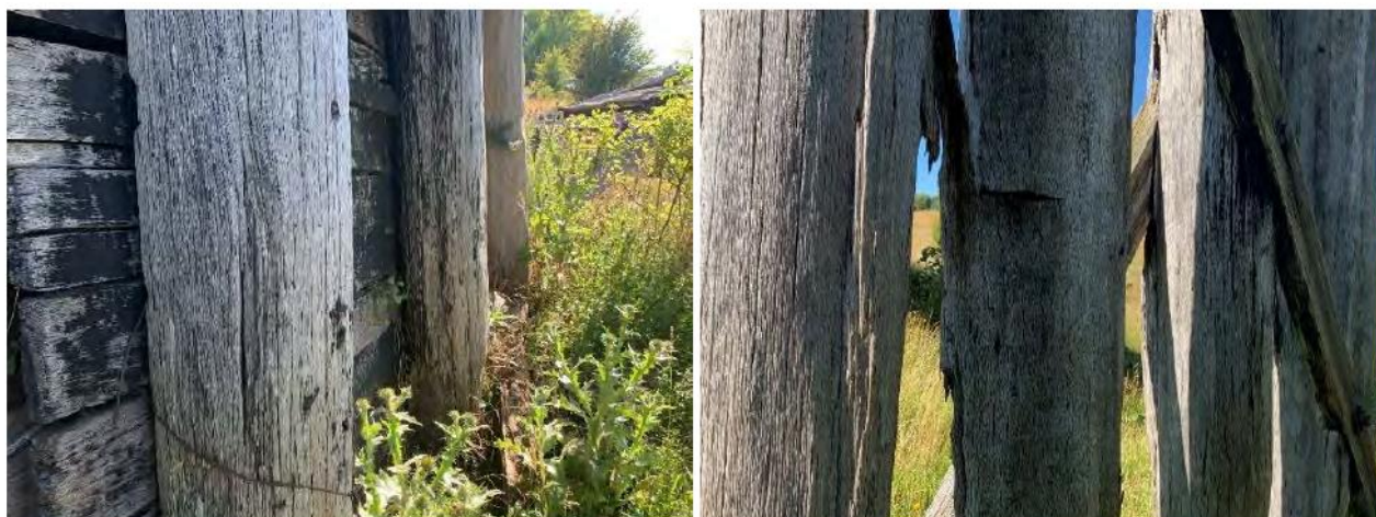
Figure 9-6: A view of two pile defects located at AB1 and PB2. The left image shows decay of sapwood forming a vertical cavity. The right image shows significant deterioration of sapwood (Peeling off).
