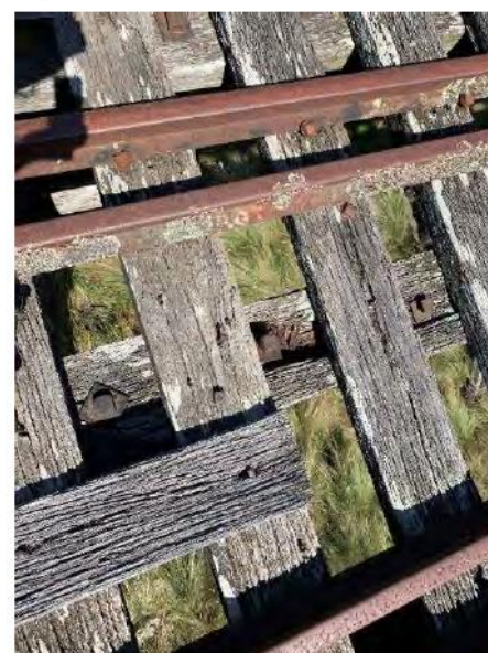
Figure 10-5: View of the walk out standing platform. Platform appears to be in poor to very poor condition with missing/failed members. This would not be safe to stand on. All timber appears to exhibit significant decay.
