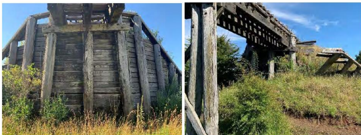
Figure 9-6: A view of two pile defects located at AB1 and PB2. The left image shows decay of sapwood forming a vertical cavity. The right image shows significant deterioration of sapwood (Peeling off).
