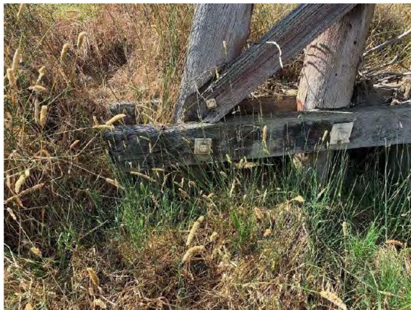
Figure 8-6: A view of a cross bracing plank connection. Plank was found to be in very poor condition as the end has completely decayed away to the connection point. Timber wales were found to be in poor condition with significant water stains and decay present throughout.
