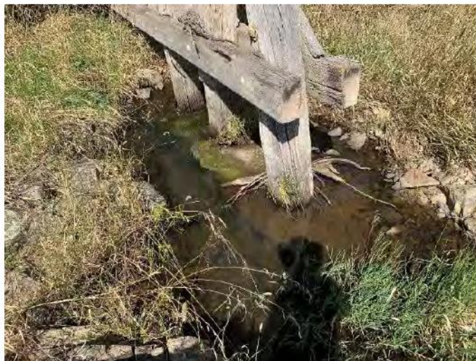
Figure 8-3: General view of pile bent 3 bearing on a concrete sill, piles were found to be in poor to very poor condition. The bottom sections of the timber piles were determined to be a ‘hotspot’ for decay and determined to be an ideal area to test using non-destructive methods, such as EPHOD® Stress Wave Technology. The timber piles were estimated to produce SWT data ranging between 300-1400 \mu s. Readings above 700 \mu s indicates that there is significant decay present and are required to be monitored. Reading of above 1000 \mu s indicate severe decay is present resulting in the member being unable to support its own dead load.
