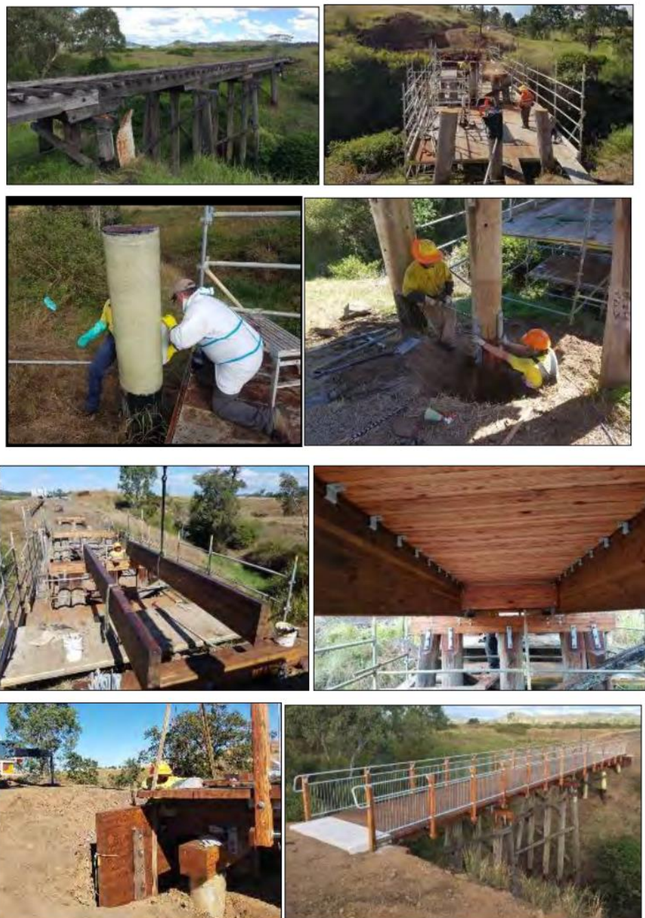
Figure 12-4: The photo series above demonstrates Option 3 type of fix that was completed on Jimmy Gully Bridge along the BVRT. The existing poor condition superstructure was removed, and the piles were repaired with high strength fibre or posted with new section. New glulam back wall, caps, girders and deck system were installed utilising a horizontal connection detail.
