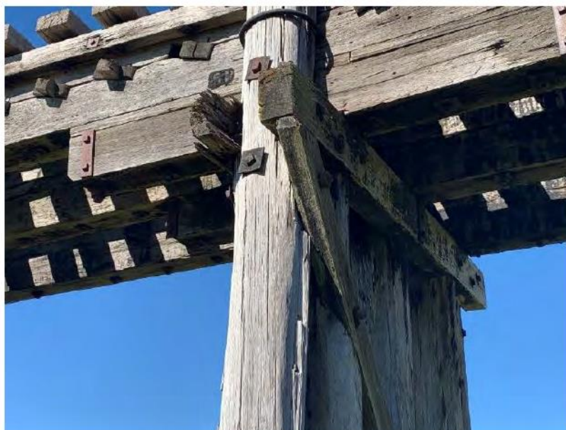
Figure 9-4: The images above show the condition of the split headstocks. The majority of headstocks were found to be in poor to very poor condition. The left member in the image above is completely decayed through the end and in very poor condition.
