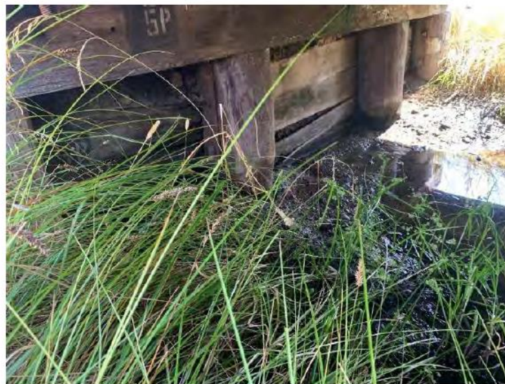
Figure 7-3: View of abutment 2, overall, in a poor condition. Sheeting planks have separated due to spiking to the pile backs in the breast wall, causing loss of fines in the approach fill material through gaps.
