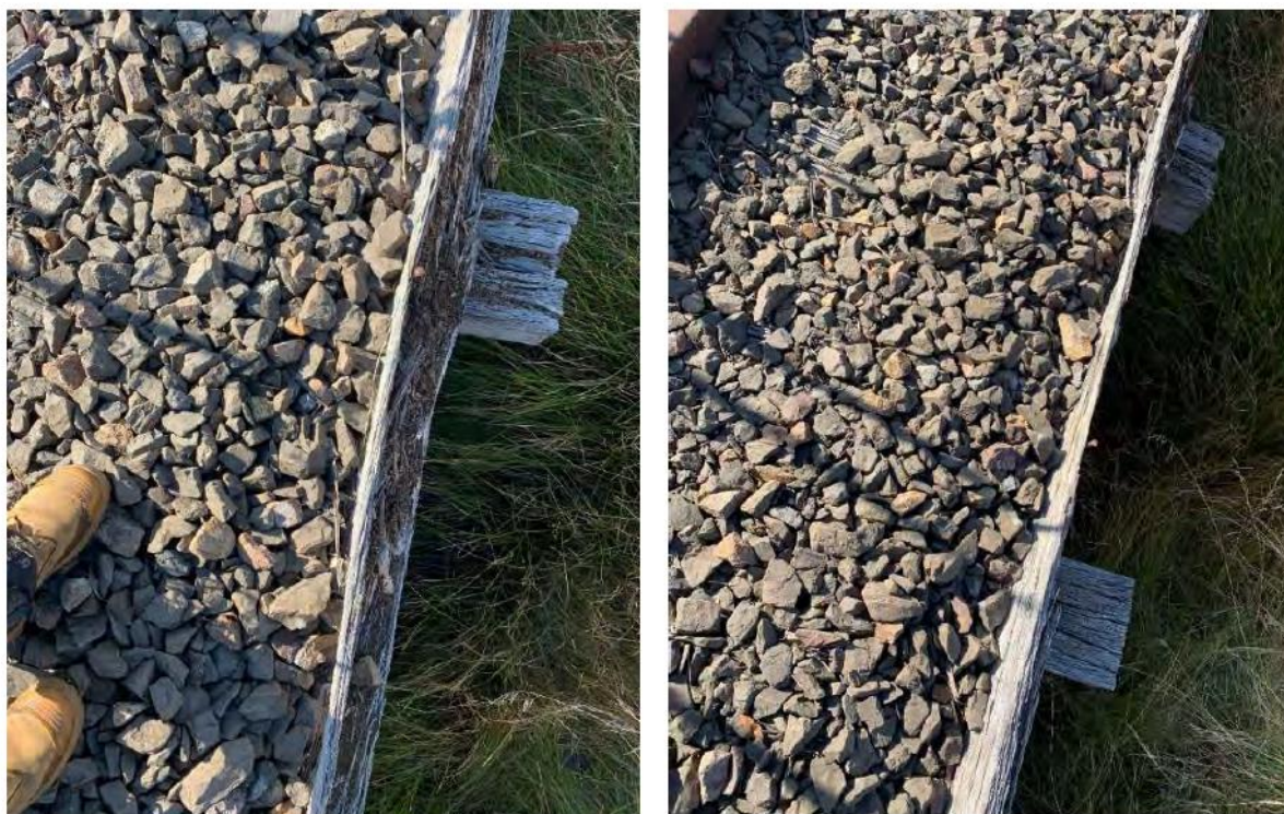
Figure 7-6: Above photos show a ballast tray side wall lengths that have completely rotted away, significantly reducing its ability to retain the ballast material.
