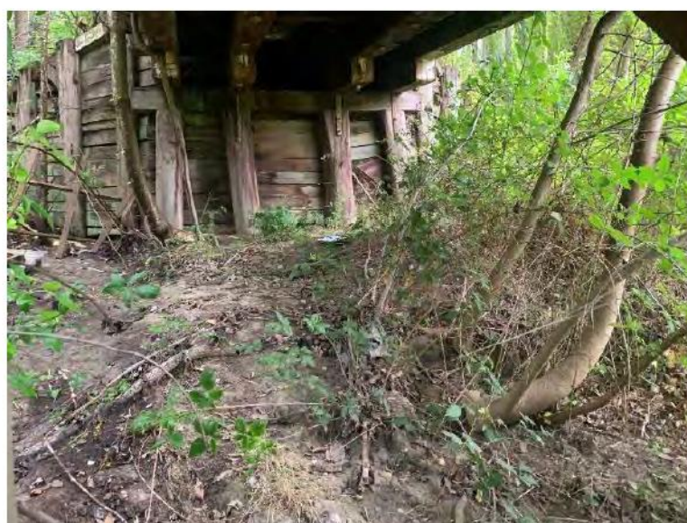
Figure 4-3: Both abutments consist of 4 timber piles, timber headstock, timber corbels and timber sheeting. It was noted that the bottom section of several piles has started to undergo decay. Note abutment sheeting is rotted and failing. Timber pile and sheeting wing walls present on both sides of each abutment. Once the moisture content in the timber elements reaches 22%, decay causing fungi are activated and the decay process begins. Large trees need to be cleared as their root systems apply lateral pressure on the substructure elements as will the branches and trunks on super structure elements.
