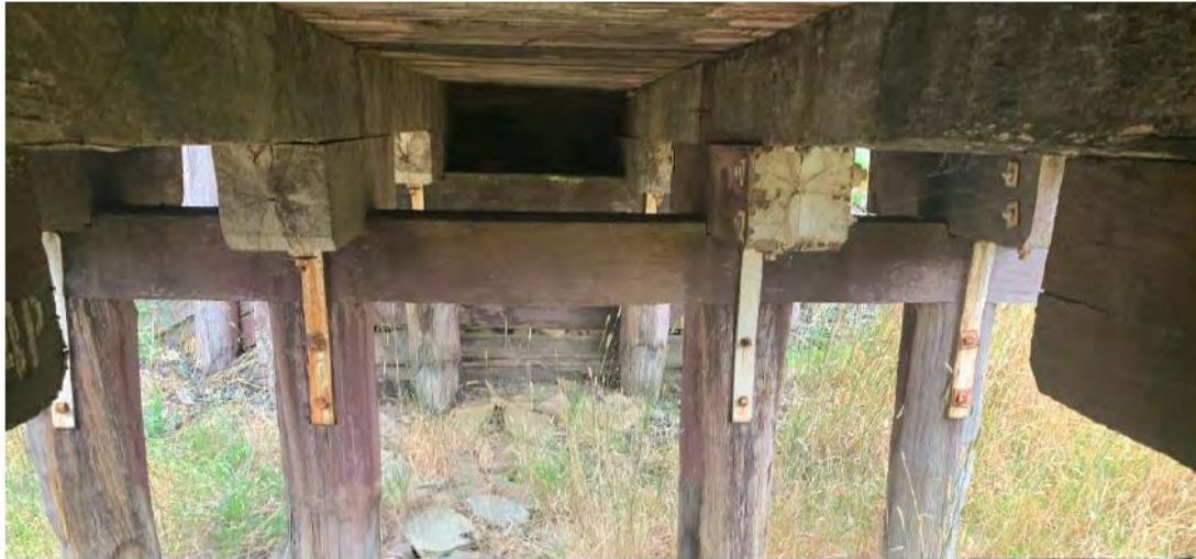
Figure 5-4: View from in between internal girders, all girders were found to be in fair condition with no major deterioration present. Corbels and bent caps were found to be in fair to poor condition throughout with evidence of minor decay present. Brief NDT testing was completed using non-destructive methods, such as EPHOD® Stress Wave Technology. Refer to Appendix A for more information of this type of testing method. Readings for girders were found to be between 300-500µs, Corbels – 400-100µs and caps 300-800µs. This is the time taken for the compression wave to travel across the section of the member tested. This was recorded on most elements and aids in verifying the condition of the elements. The pile tops are in better condition due to the use of horizontal connectors with side plates.
