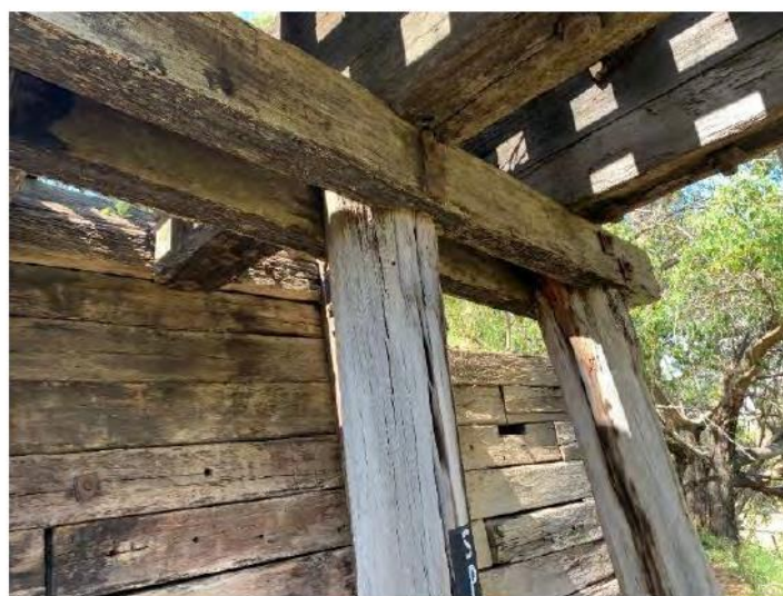
Figure 10-4: The images above show the condition of the split headstocks and the abutment breast wall. The headstocks were found to be in poor to very poor condition, exhibiting significant decay. The breast wall is in poor condition with missing members and weathered elements with splits and cracking throughout. Note: major vertical crack down middle pile exposing bright wood and accelerating decay. Typically, these decay cracks are initiated by fastener systems
