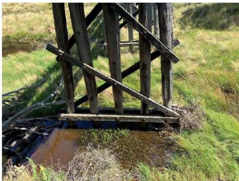
Figure 10-3: Significant decay is present on all piles in above image. Large decrease in pile cross-section on the bottom end of the piles located in the river (Body of water). Debris is caught up in the wales and surrounding areas of pile bents. It is recommended that deteriorated sapwood be removed appropriately.
