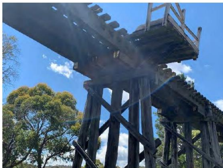
Figure 10-5: View of the walk out standing platform. Platform appears to be in poor to very poor condition with missing/failed members. This would not be safe to stand on. All timber appears to exhibit significant decay.
