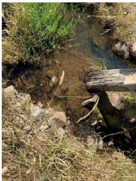
Figure 8-3: General view of pile bent 3 bearing on a concrete sill, piles were found to be in poor to very poor condition. The bottom sections of the timber piles were determined to be a ‘hotspot’ for decay and determined to be an ideal area to test using non-destructive methods, such as EPHOD® Stress Wave Technology. The timber piles were estimated to produce SWT data ranging between 300-1400 \mu s. Readings above 700 \mu s indicates that there is significant decay present and are required to be monitored. Reading of above 1000 \mu s indicate severe decay is present resulting in the member being unable to support its own dead load.
