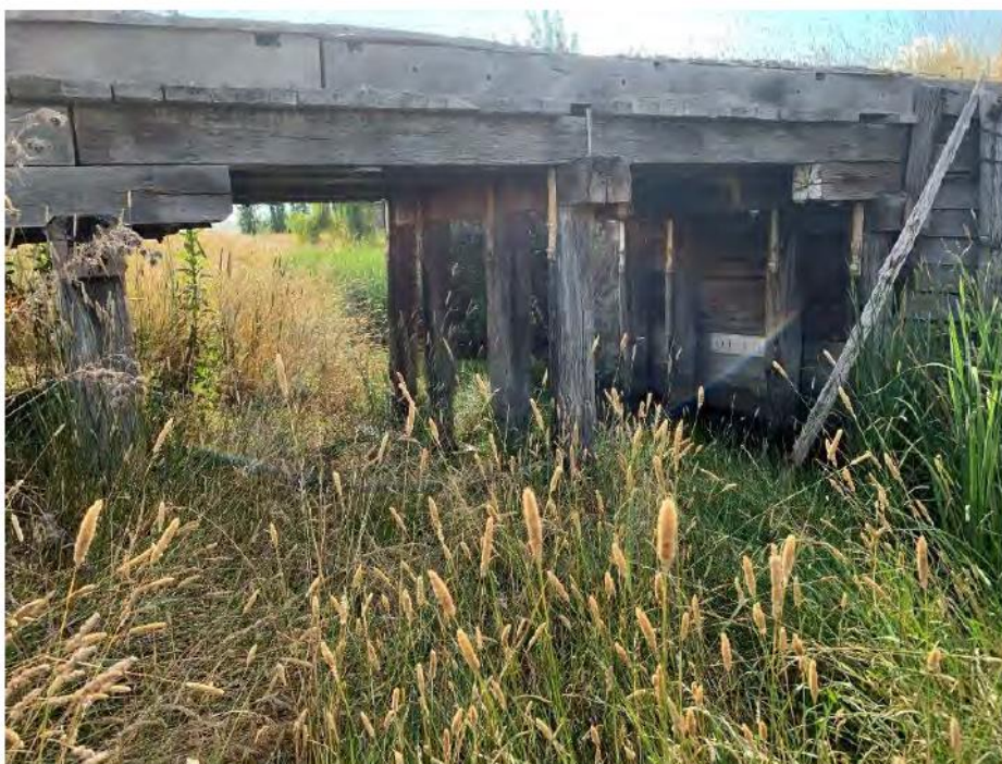
Figure 6-1: General view of Lobbs Hole Creek Bridge from the side of the bridge. The Creek that flows underneath span 1 at the time of inspection was flowing very slowly/still. The configuration of the bridge is a girder under and consists of 3 spans, 2 abutments and 2 pile bents. The span length is 3m equating to a total length of 12m. Note: abutment 1 and abutment corbels as does one of the bents.
