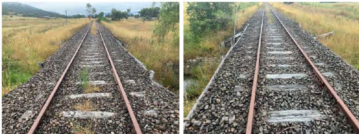
Figure 5-8: Top view of rock ballast looking in opposite directions. The rock ballast was found to be in fair condition with no major erosion present, no holes were found in bridge decking. Transoms were found to be in fair to poor condition with moderate deterioration and decay found.
