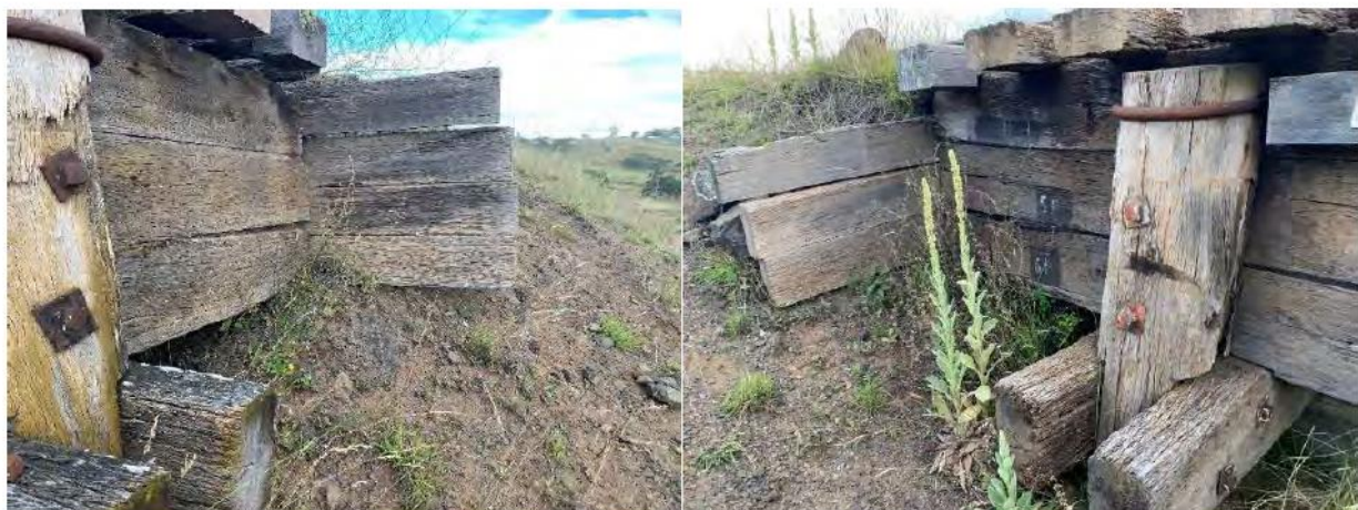
Figure 11-4: The images above show the condition of the breast wall at AB2. The abutment sheeting was found to be in fair condition with minor decay of the sapwood present. The headstock ends were in poor condition with decay and cracking present.
