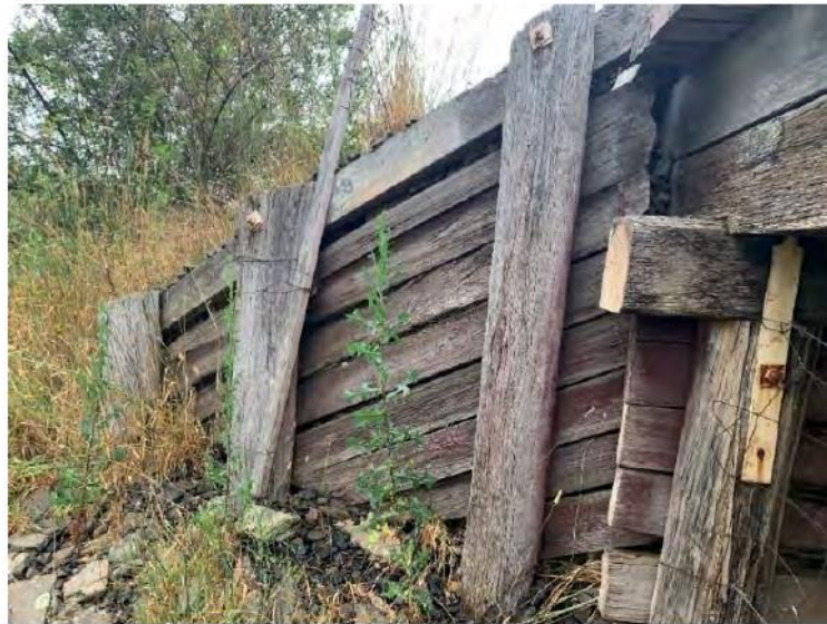
Figure 5-6: A view of abutment wingwall. The wingwall was found to be in fair to poor condition with minor deterioration present throughout all components. Minor deformation was present at top of wall due to bearing load of ballast.
