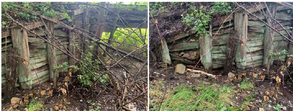
Figure 4-8: The timber wingwalls have undergone significant deterioration with timber sheeting completely rotted and failing in several locations. Due to this the walls' ability retain the approach fill material is poor leading to erosion and excessive loading.
