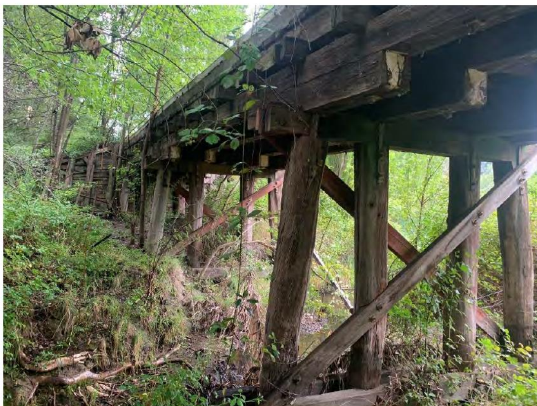
Figure 4-1: View of Guises Creek Bridge from end 1. The timber bridge is 3 spans long and approximately 24m metres long (8 metre spans). Note at all bents each girder has a corbel. Note that the corbels and girders are dimension timber when typically, they will be round log. At the time of inspection there was only water underneath span 2 with an approximate depth of 0.5m. There is a large amount of vegetation growth around the timber bents which keeps the moisture content of the timber high. When the moisture level in the timber is above 22%, decay-causing fungi can start to grow; when the moisture content drops below this level, the fungi become dormant, and decay will be arrested until the moisture content rises again. It is noted that a resin treatment has been used to fill existing cavities in majority of the girders. Note the rounded drip edge on the corbels. A positive detail. However, plenty of poor detailing vertical fasteners originating from the top of the girders are in use.
