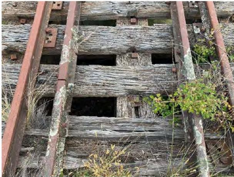
Figure 11-7: View of the bridge open deck, transom sleepers were found to be in poor to very poor condition with significant decay, cavities and severely damaged members present throughout. It was noted that the vertical connections to the top girders were seen to funnel moisture and increase the moisture content present in both elements causes significant decay. When the moisture content exceeds 22%, timber consuming fungi are activated, and the decay process begins. Top girders were found to be in poor to very poor condition.
