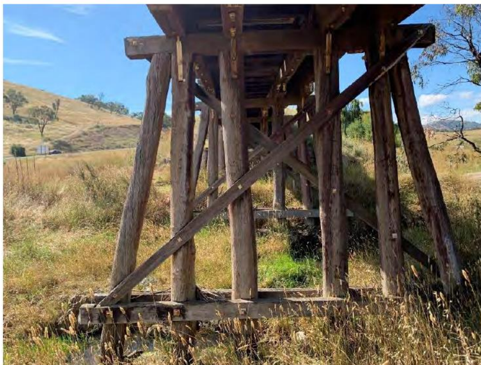
Figure 8-2: View of the typical timber pile bents configuration. The bents comprise of 6 driven piles (4 Plum piles directly under the girders and 2 batter piles on either side). Pile bent 2 and 3 are supported by cross bracing and timber wales at the bottom of the bent. Pile bent 3 was constructed on a concrete footing. The two abutments do not contain the cross bracing and wales. It was noted that the bottom section of several posts and timber cap wales have started to undergo decay. This can be expected due to the timber posts bearing directly on the concrete footing which typically has a high moisture content. Over time the timber post undergoes capillary action and draws up the moisture like a ‘straw’. Once the moisture content in the timber elements reaches 22%, decay causing fungi are activated and the decay process begins. Overall, the timber bents were found to range from fair to very poor condition.
