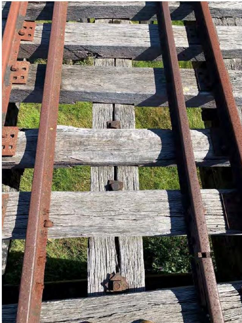
Figure 9-8: Top view of bridge surface, found to be in poor to very poor condition due to major vertical crack through the middle girder and major decay present in all other girder lengths. Vertical connections expose the bright wood to weathering and funnel watering, this leads to accelerated decay and higher moisture content. Transoms appear to be in fair to poor condition with no major decay or defects present. Note the smaller guard inner guard rail on this open deck railway bridge
