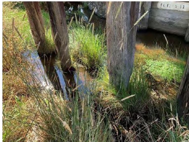
Figure 6-3: A view of Bent 2 shows the timber piles were driven into the creek. Significant sapwood decay is present in the lower length of each pile as seen by the noticeable change in cross section. This is seen as a length that is subject to temporary exposure to moisture which causes accelerated decay compared to constant saturation. Once the moisture content exceeds 22%, timber consuming fungi are activated, and the decay process begins. Refer to Figure 3-2 for a detailed description of how and where the decay occurs due to these vertical bolts.
