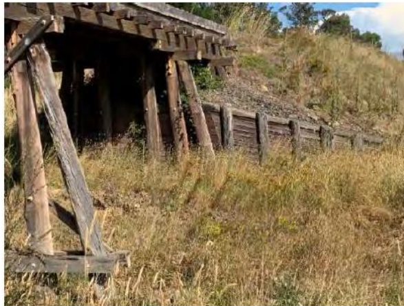
Figure 8-4: The images above show the condition of the breast wall at PB1 & 4. The left photo shows the breast wall at PB1 to be poor to very poor condition with significant decay in timber elements present, surrounding overgrown vegetation and erosion of back fill material. The right image shows the breast wall at PB4 to be in fair to poor condition, it was noted that the back fill material had forced the wall to “lean” forward. Note: Severely decayed batter pile at PB3.
