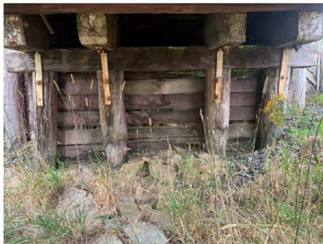
Figure 5-4: View from in between internal girders, all girders were found to be in fair condition with no major deterioration present. Corbels and bent caps were found to be in fair to poor condition throughout with evidence of minor decay present. Brief NDT testing was completed using non-destructive methods, such as EPHOD® Stress Wave Technology. Refer to Appendix A for more information of this type of testing method. Readings for girders were found to be between 300-500µs, Corbels – 400-100µs and caps 300-800µs. This is the time taken for the compression wave to travel across the section of the member tested. This was recorded on most elements and aids in verifying the condition of the elements. The pile tops are in better condition due to the use of horizontal connectors with side plates.
