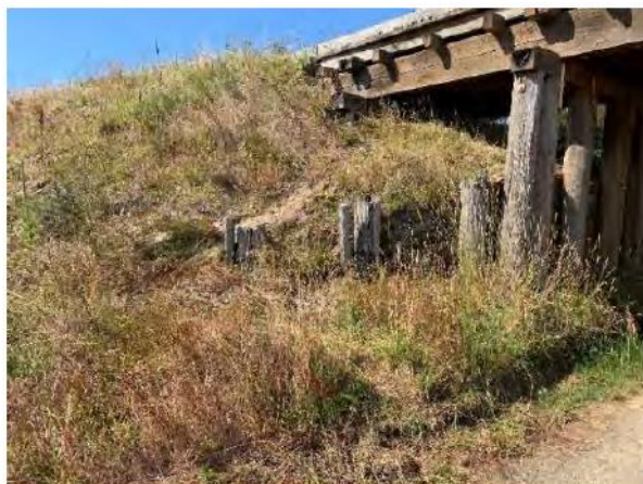
Figure 8-4: The images above show the condition of the breast wall at PB1 & 4. The left photo shows the breast wall at PB1 to be poor to very poor condition with significant decay in timber elements present, surrounding overgrown vegetation and erosion of back fill material. The right image shows the breast wall at PB4 to be in fair to poor condition, it was noted that the back fill material had forced the wall to “lean” forward. Note: Severely decayed batter pile at PB3.
