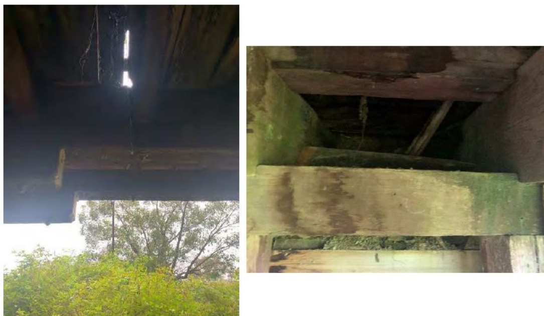
Figure 4-7: The photo on the left shows a failed deck plank from below. The photo on the right shows another failed deck plank located above the abutment. Decking failure causes the above rock ballast to erode and elements below experience excess weathering and load. These planks will require replacement before the bridge can be reopened for pedestrian and cycle use.
