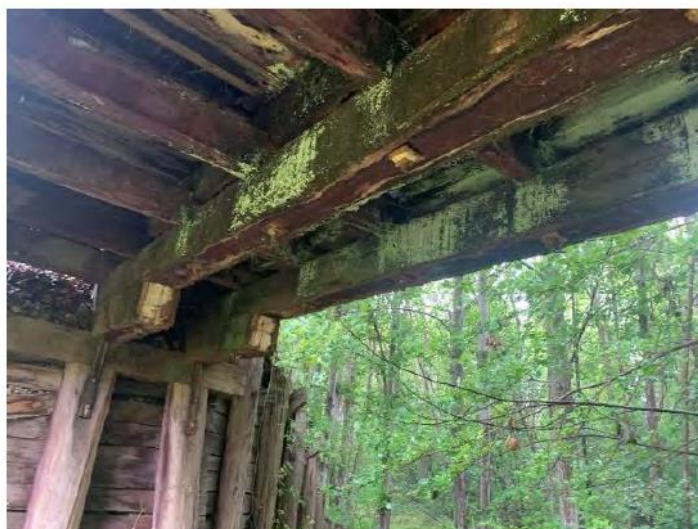
Figure 4-6: View of 2/4 girders. Consists of 4 girder lines which are double stacked with the top girder serving as a lateral bearer beam end stabilizer as well increasing the elevation of the ballast tray floor. All girders exhibited major water stains and decaying fungal growth. Girders were found to be in poor to very poor condition.
