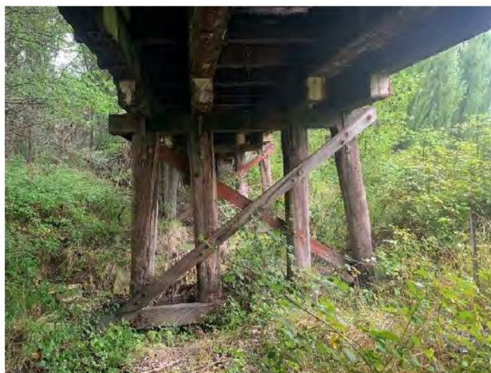
Figure 4-2: View of the typical timber pile bent configuration. The bent is comprised of 4 driven piles, single timber head stocks and corbels. The bent is also supported by a double cross bracing system with sashes at halfway and timber wales at the bottom. Overall, the timber bents were found to be in a poor to very poor condition. Note the surface brown rot fruiting bodies on the faces of some of the cross braces -orange brown colour.
