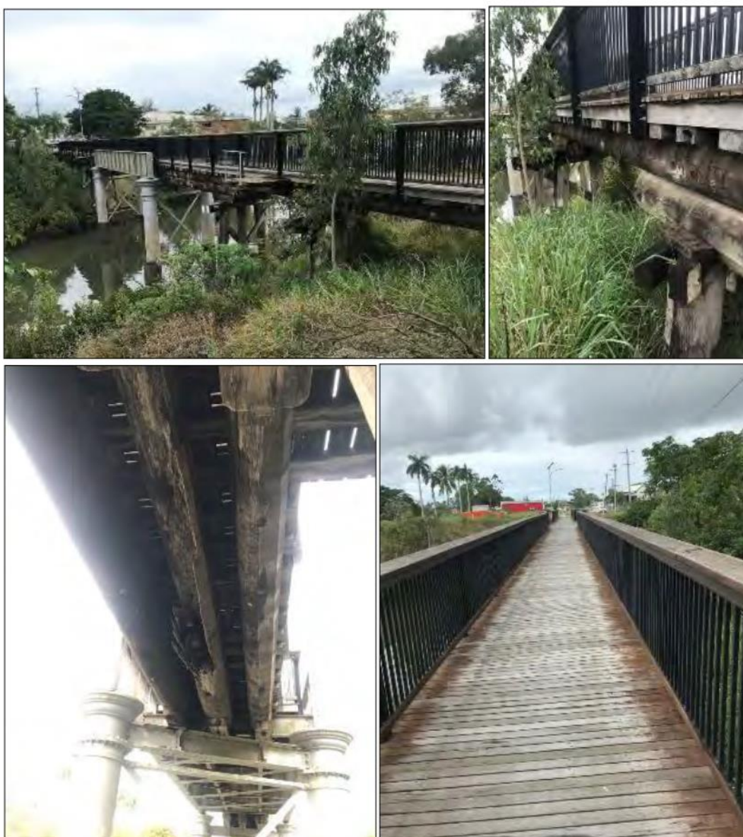
Figure 12-2: The above photo series demonstrates a similar repair to Option 1 type of refurbishment (build off existing railway bridge) used for the construction of a pedestrian bridge in Bundaberg CDB. The existing railway bridge was left un-touched and a new hardwood deck system with handrails was installed. Six 100mm x 250mm timber joists were placed on top of the existing transoms (rail ties) with a 38-50mm thick hardwood deck installed on top. This option will likely be the lowest cost but also carries the shortest expected lifespan. As seen in the bottom left photo above, one of the girders has failed and fallen out creating a 'weak' point along the bridge. Due to a high residual capacity of timber and the continuous joists, a complete failure of the bridge (span) hasn't occurred yet but is only a matter of time unless extensive maintenance is undertaken.
