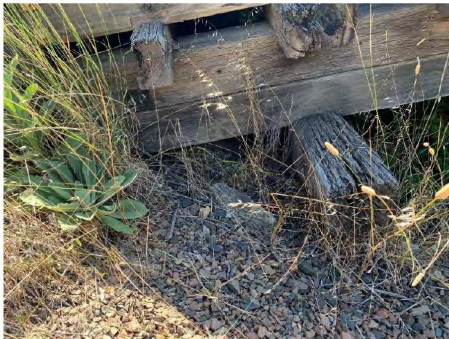
Figure 8-8: View of Abutment cap and spacing logs, cap is in very poor condition due to the large cavity and significant decay present at both ends. Spacing members were found to be in fair to poor condition with sapwood decay and cavities present.
