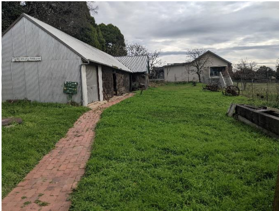
Figure 5 - View of rear of site, existing shed to the left
