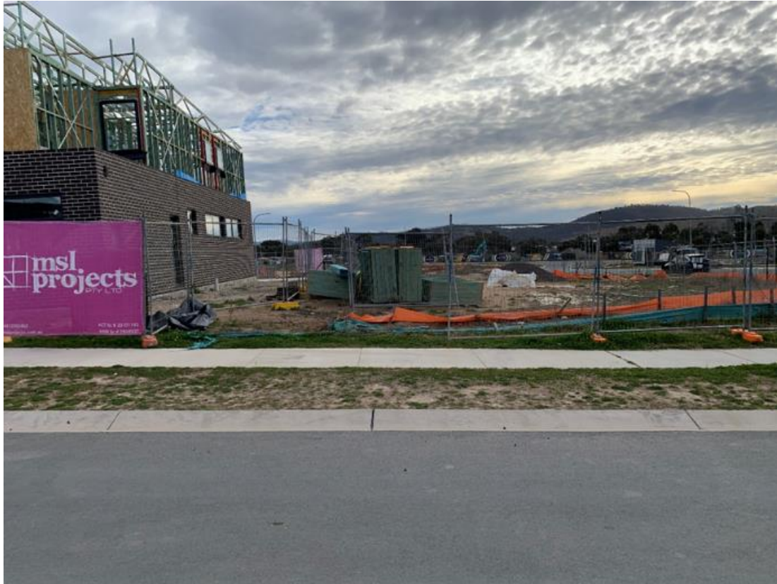
Figure 8: Access for Lot 339 off Tassel Terrace
