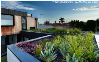
Example of semi extensive roof garden
