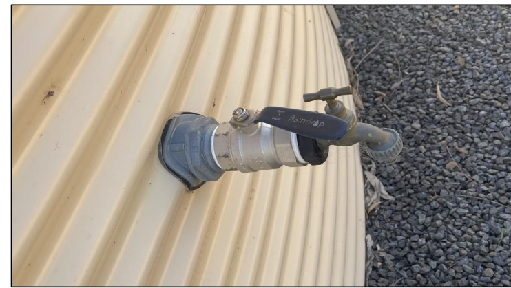
Figure 21 – Tap fitting showing 30,000L of dedicated firefighting water below.
