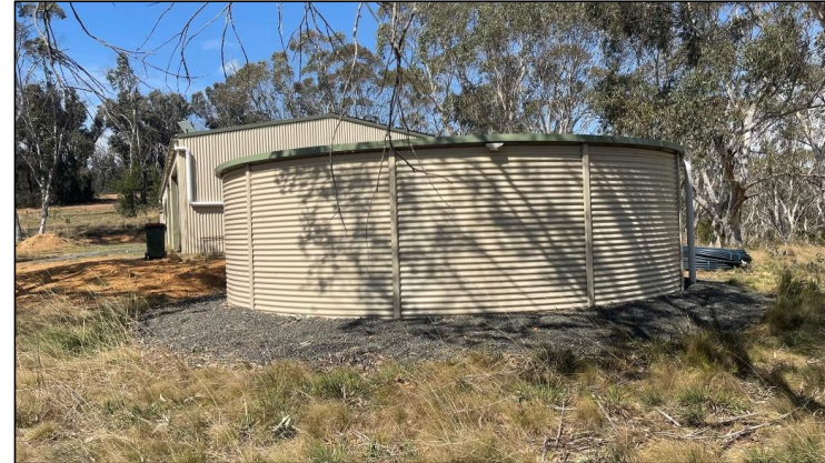
Figure 20 – Second interconnected 109,000L metal water tank with Stortz fitting.
