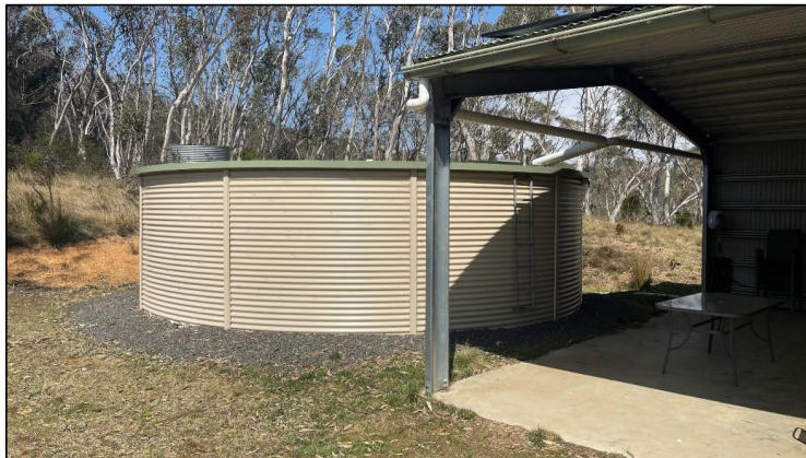
Figure 19 – Existing 109,000L metal water tank fed from shed roof. (McGregor, 2023)
