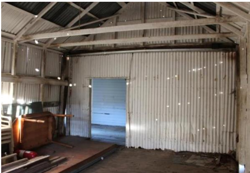
Figure 10 – Image inside western portion of T -shaped shed (image taken 2021-22)
