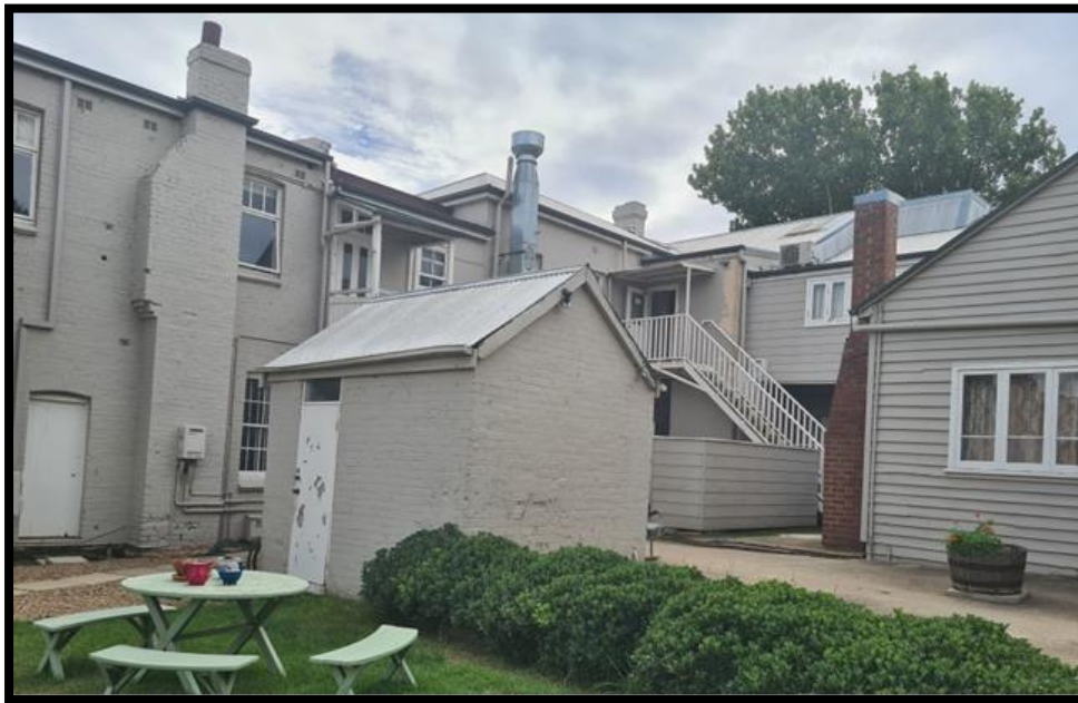
Figure 13 – small brick shed where roof awning proposed
