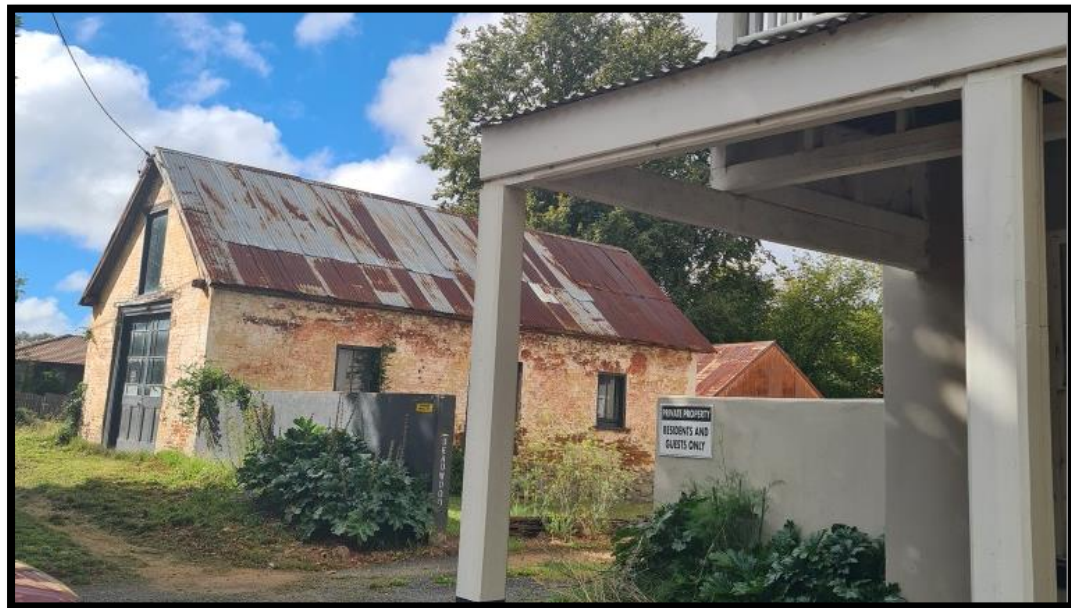
Figure 3 – Stables with awning of Albion Hotel in foreground
