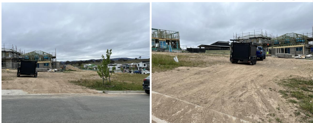
Figures 3 and 4: Site photos
