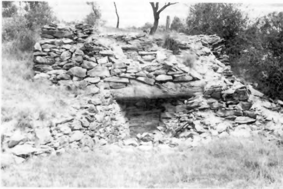
Moses Morley's 1870s kiln on Stringybark Hill south of Queanbeyan. The massive tree trunk supporting the upper part of the kiln's front wall probably helped to stabilise it during the burning process. The front walls of kilns tended to bulge outward with the intense heat. (Photograph by author).
