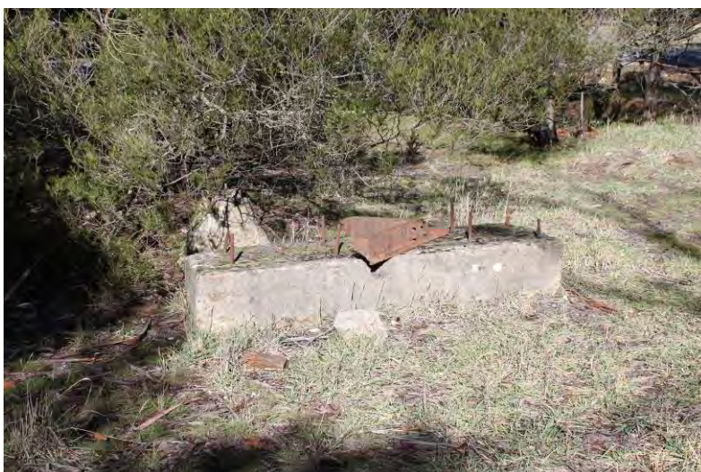
Machinery footing
