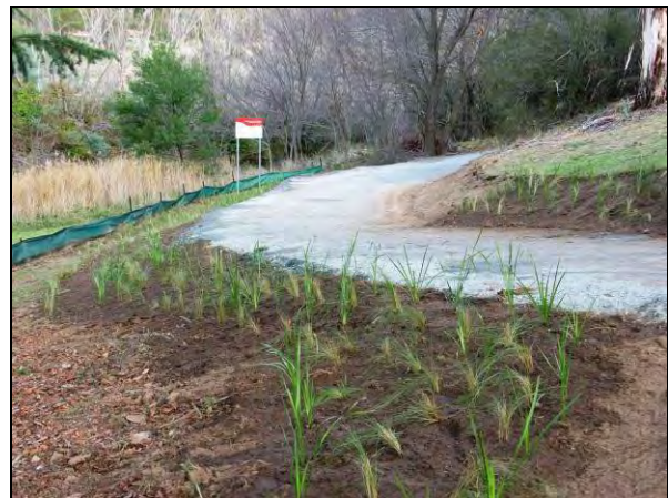
Revegetation and path construction
