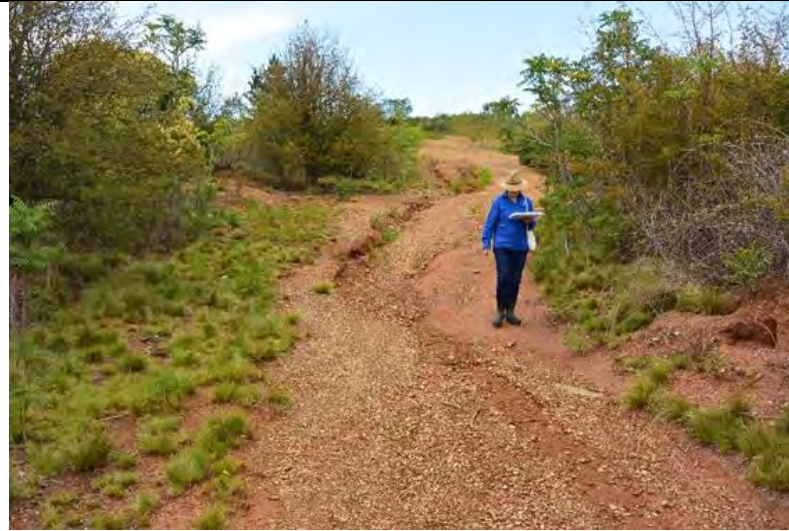
DSC 3781: Eroding trails leading into the quarry site
