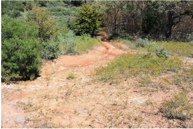
DSC 3833: Sheet and rill erosion across the site
