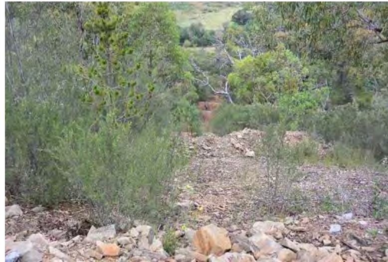
DSC 3767: Erosion control earthworks
