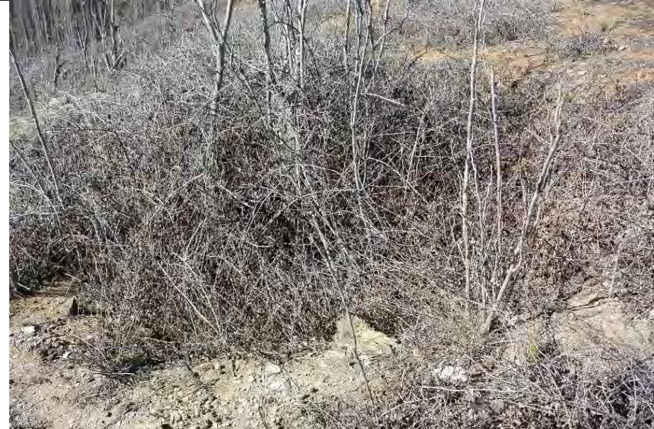
DSC 3012: Partially obscured mine adit creating safety hazard
