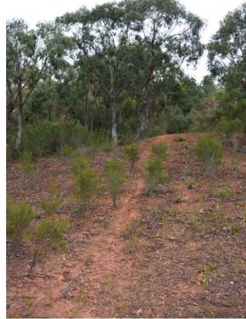
DSC 3775: Tracks eroding bank freeboard
