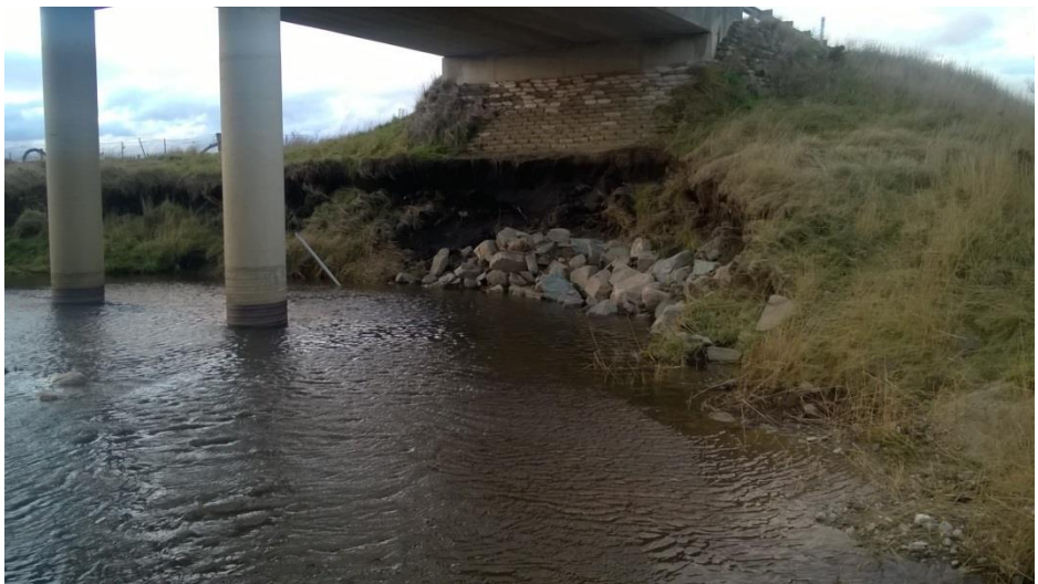
Figure 3 – June 2016 Flood Damage – Deep Creek Bridge
