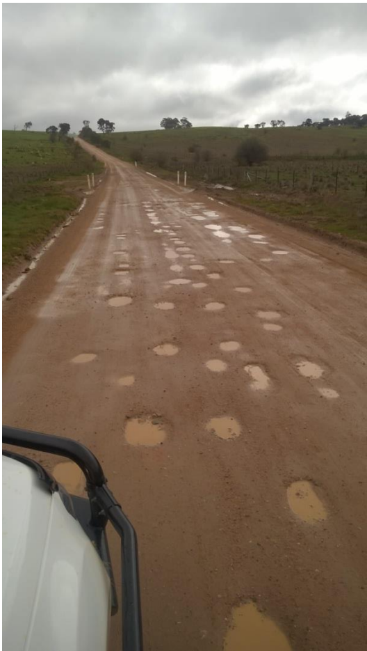
Figure 1 – Unsealed Road Potholed Pavement - Potholes
