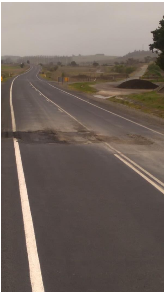
Figure 2 – Sealed Road Pavement – Pavement Failure
