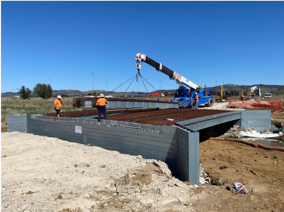
Works on the Halfway Creek bridge replacement.
