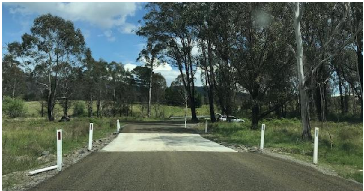
The bridge on River Forest Road was replaced during 2022-23.
