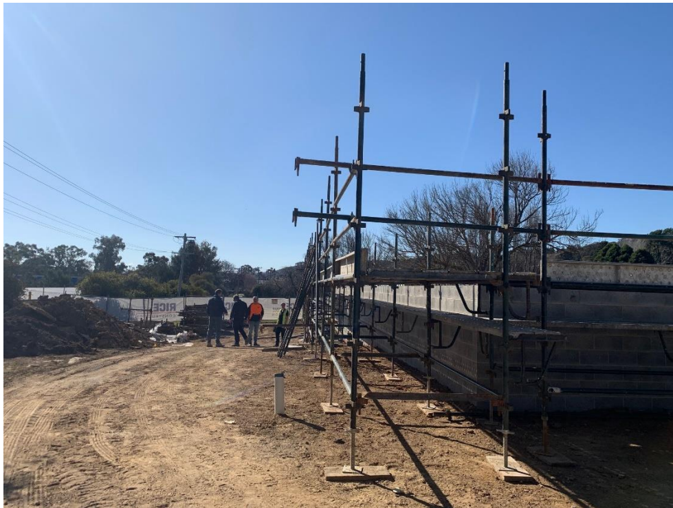
Construction commenced on the Wright Park amenities building.
