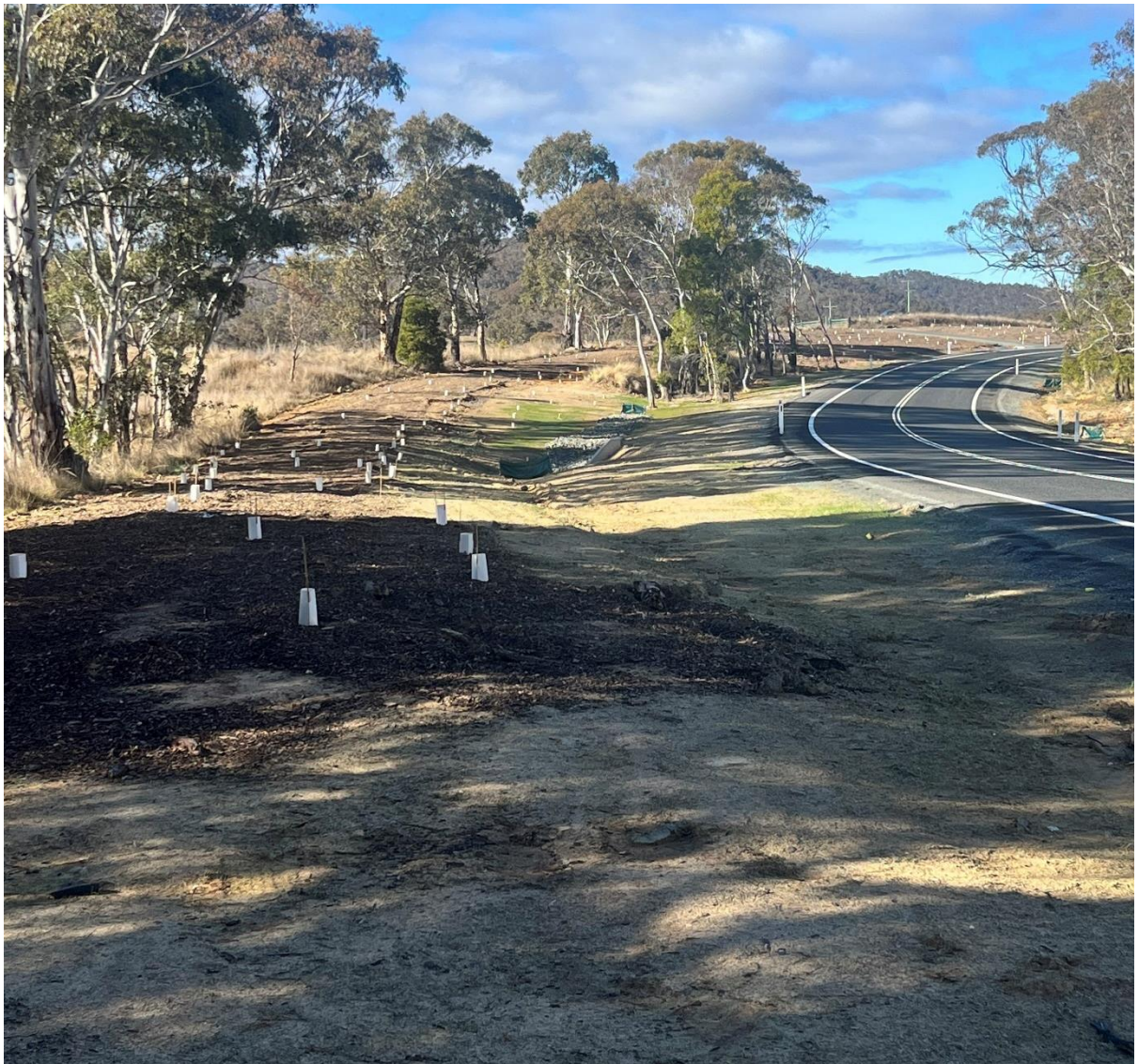
Tree planting along a reconstructed section of Captains Flat Rd.
