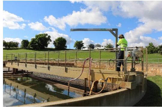
Photo 24: Sewage Treatment Plant
