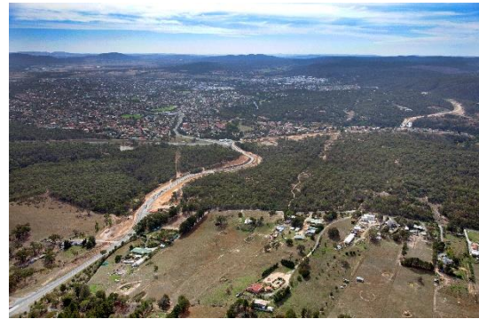
Photo 20: Old Cooma Road realignment for Googong
