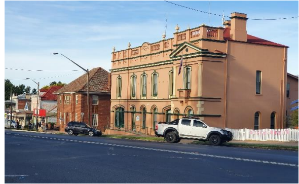
Photo 26: Braidwood office building
