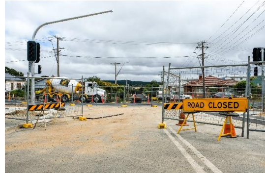
Photo 21: Uriarra Road and Ross Road intersection
