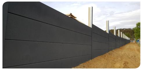
Image of partially completed noise wall along Ellerton Drive, transparent panel to be installed above concrete panels.
