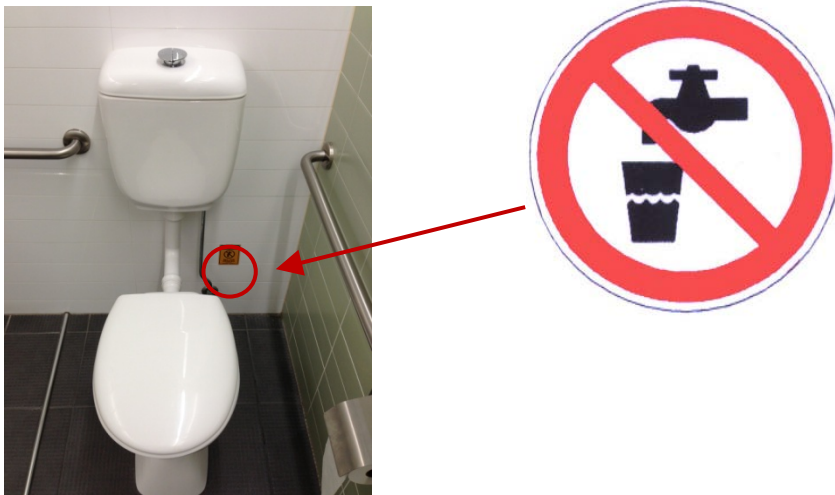
Figure 7: Example of signage for the toilet
