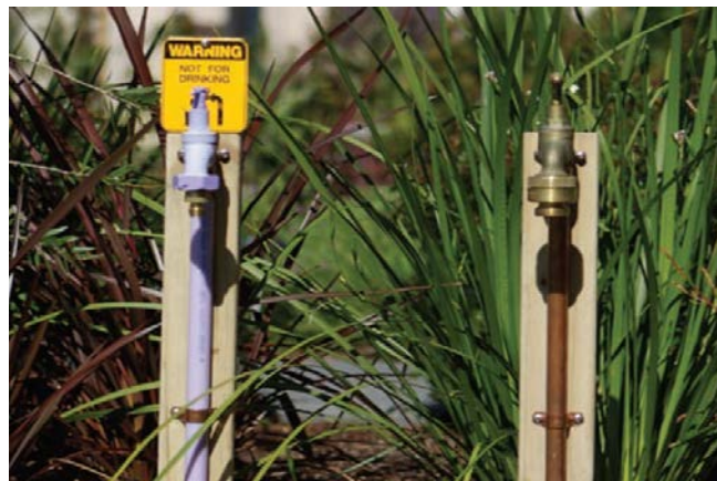
Figure 8: Outdoor recycled water tap (left) and drinking water tap (right)
