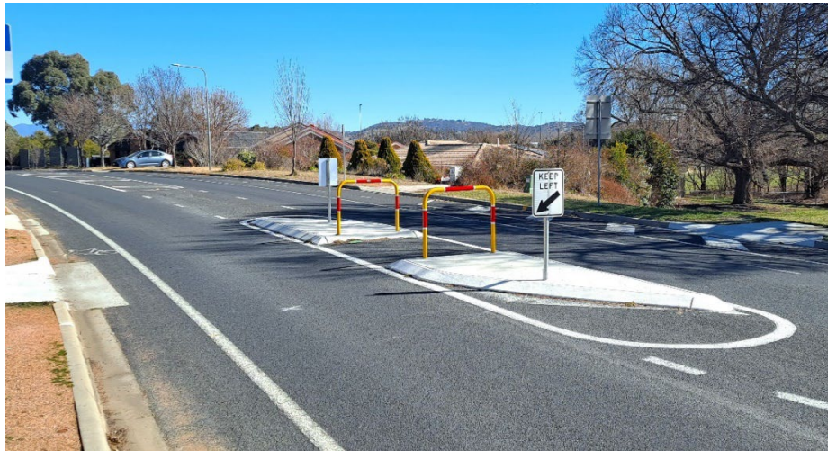
Figure 2: Example midblock pedestrian refuge island.
