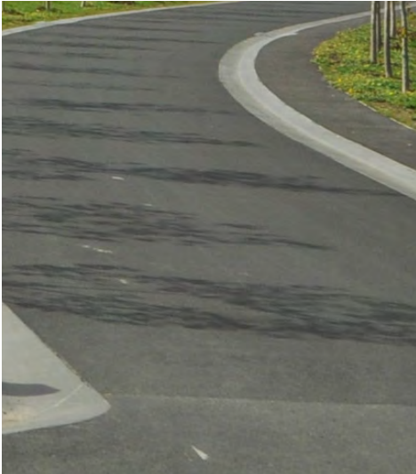
HOTMIX BLACK ASPHALTIC CONCRETE WIDE CONCRETE EDGING
