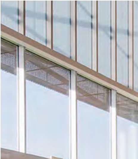
GLAZING / TRIMS FIXED AND OPERABLE ALUMINIUM GLAZING POWDER-COATED WHITE
