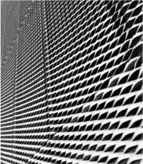
EXPANDED MESH CLADDING EXPANDED MESH SCREENS PANELS FIXED TO PAINTED CFC SHEET COLOUR - WHITE
