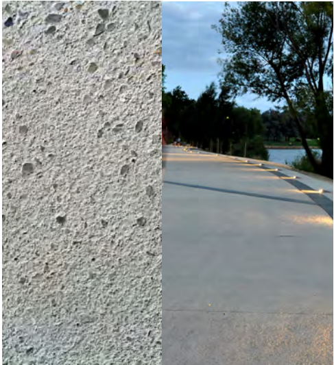
INSITU CONCRETE NON-SLIP FINISH LIGHTLY EXPOSED
