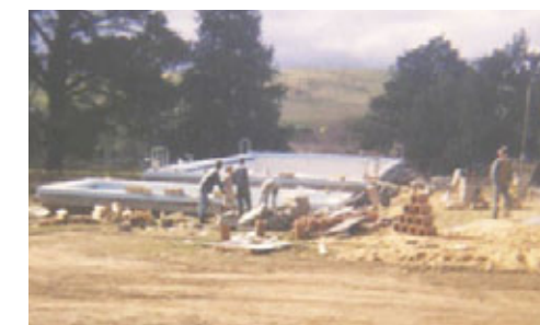
C View C- Braidwood Swimming Pool under construction Note:- pool built above existing levels (levels raised)
