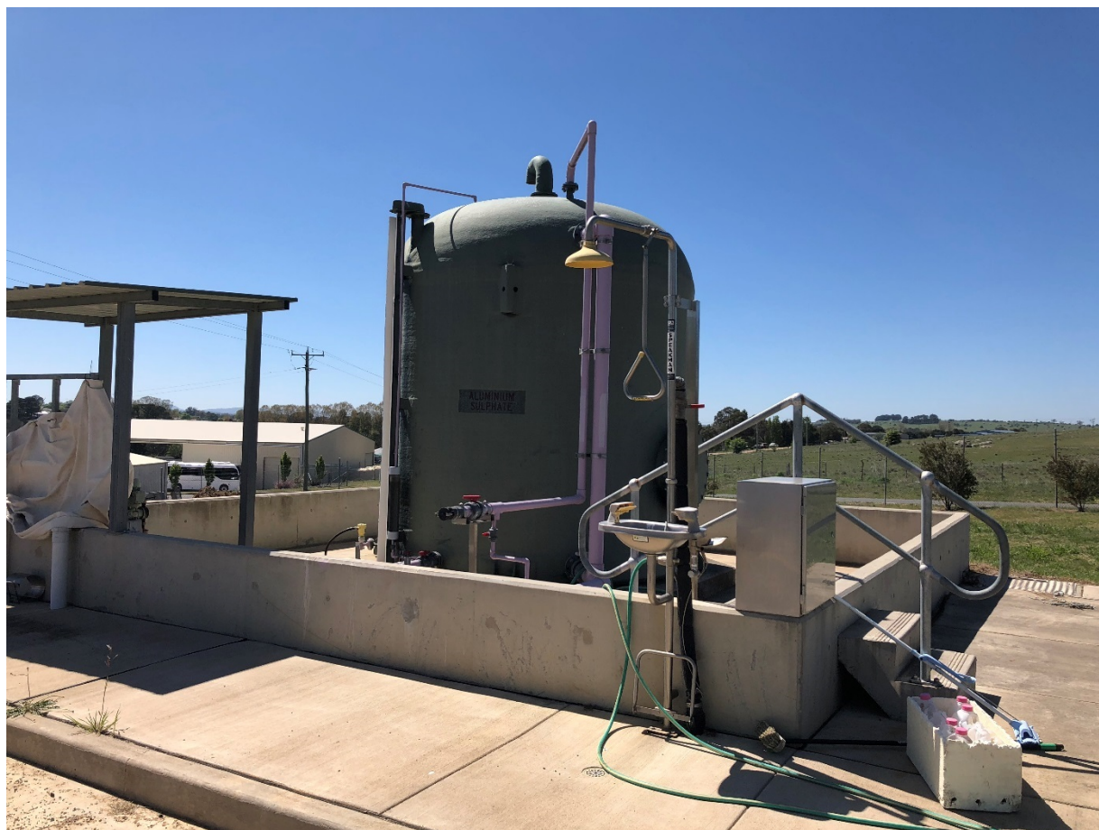
Figure 14 - 5: Braidwood STP – Chemical Storage Alphos for Phosphorus Removal
