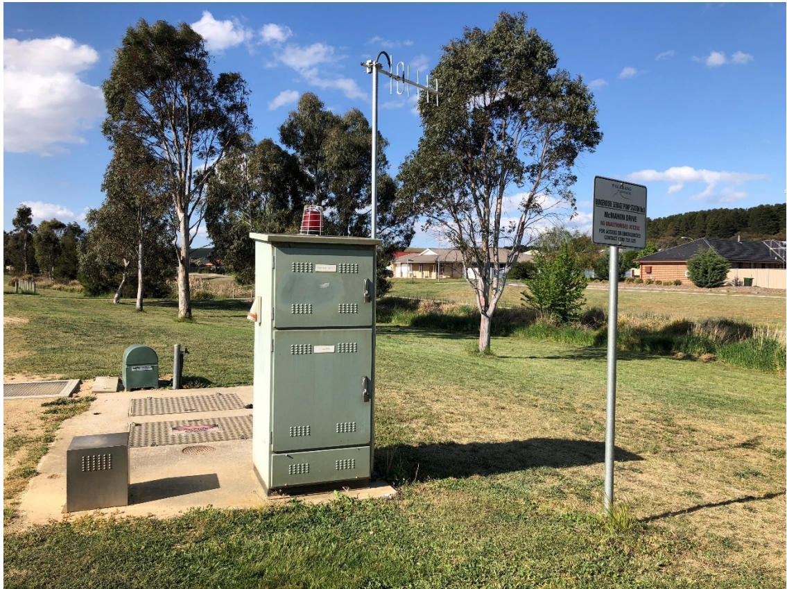
Figure 6 - 9: Typical Installation for Visible Alarm Light
