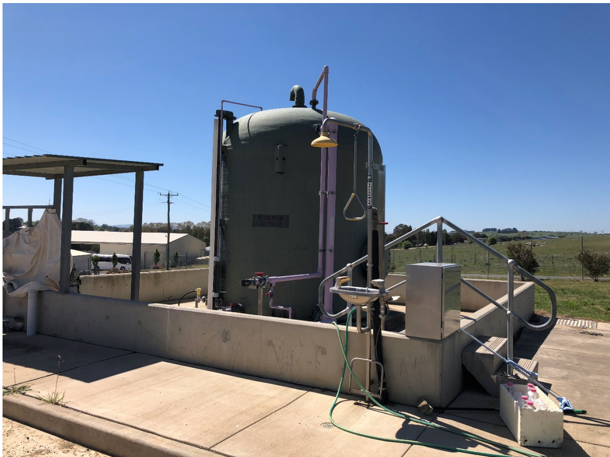
Figure 6 - 10: Typical Chemical Storage Arrangement for QPRC STPs
