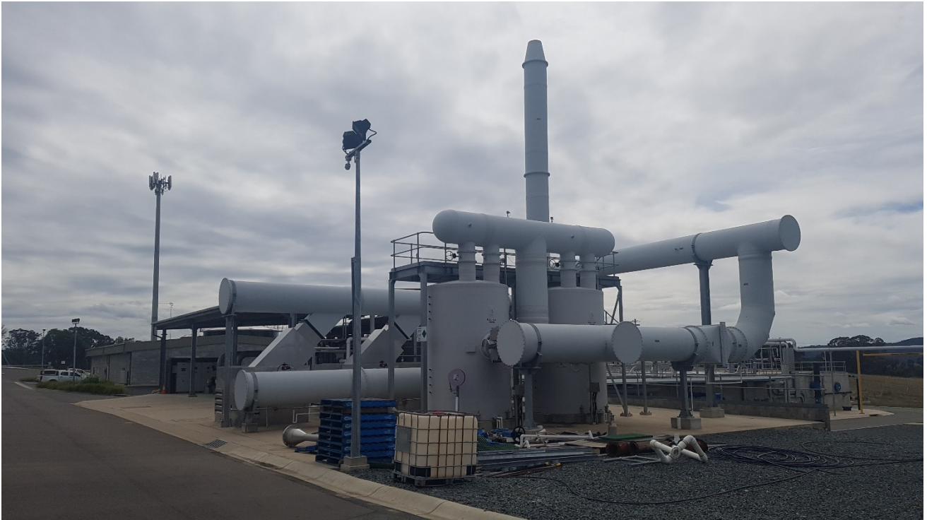
Figure 15-6 Googong WRP – Odour Control Facility
