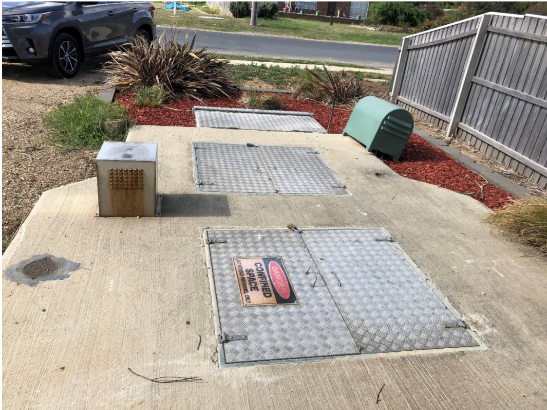
Figure 13 - 11: Activate Carbon Unit Located at SPSs
