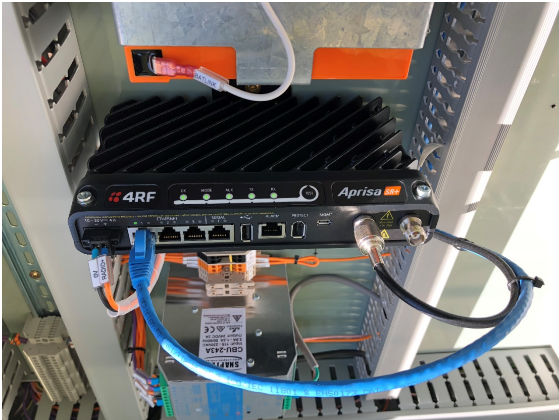
Figure 6 - 4: Telemetry Remote Terminal Unit (RTU)
