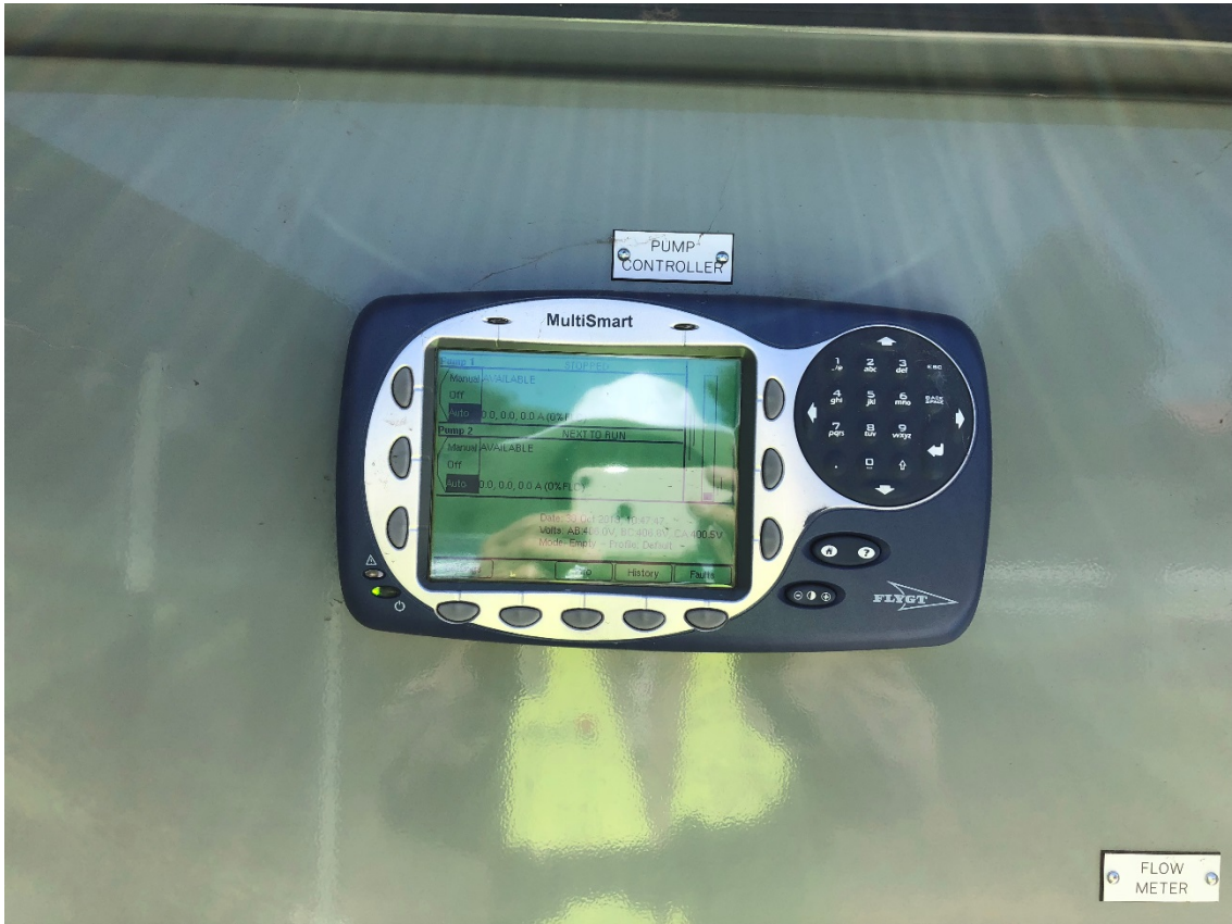
Figure 6 - 4: Telemetry Remote Terminal Unit (RTU)
