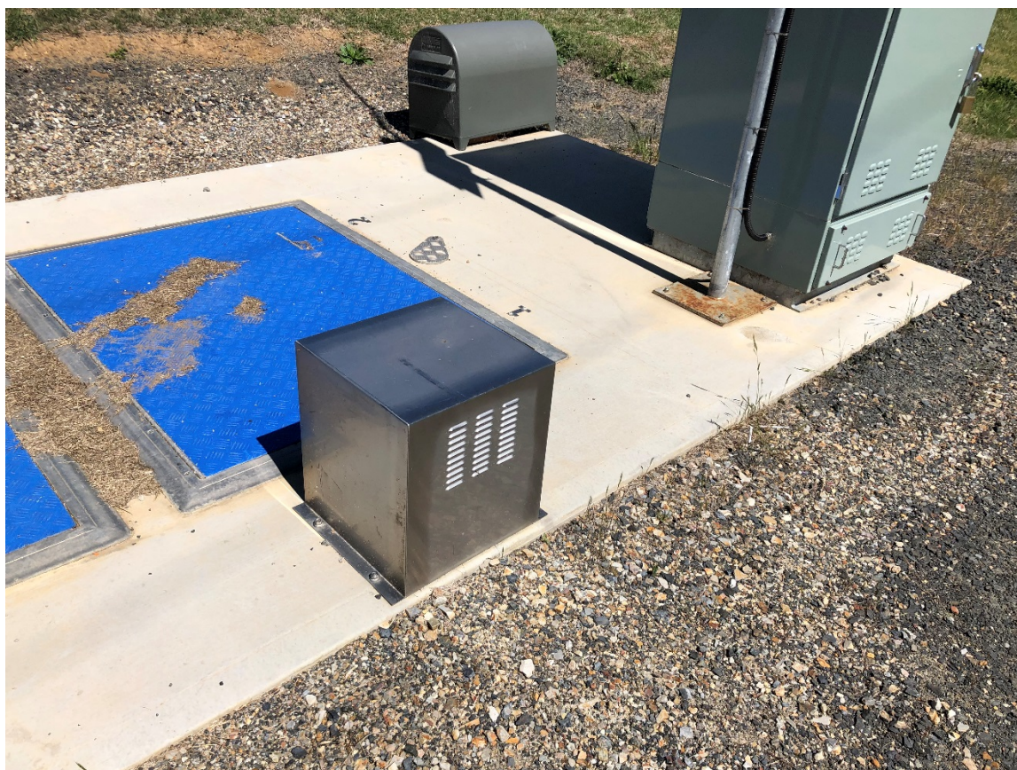
Figure 14 - 7: Activated Carbon Unit Located at SPSSs
