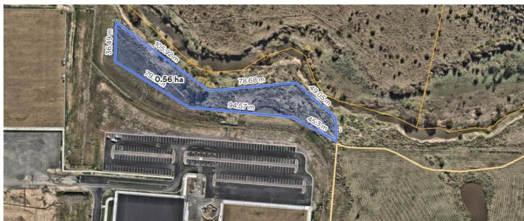
Figure 4: Regional Sports Complex on Environa Drive
