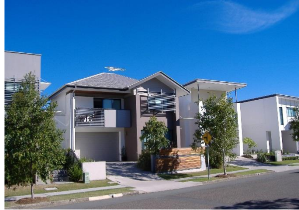
Garage set back to rear laneway
