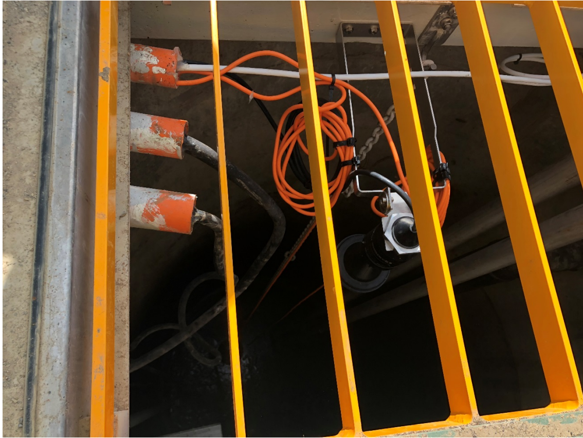
Figure 6 - 9: Typical Installation for Visible Alarm Light
