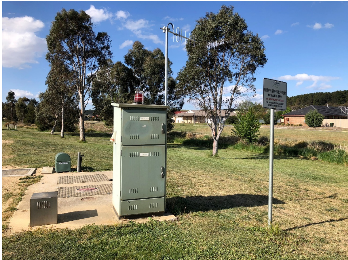
Figure 6 - 9: Typical Installation for Visible Alarm Light
