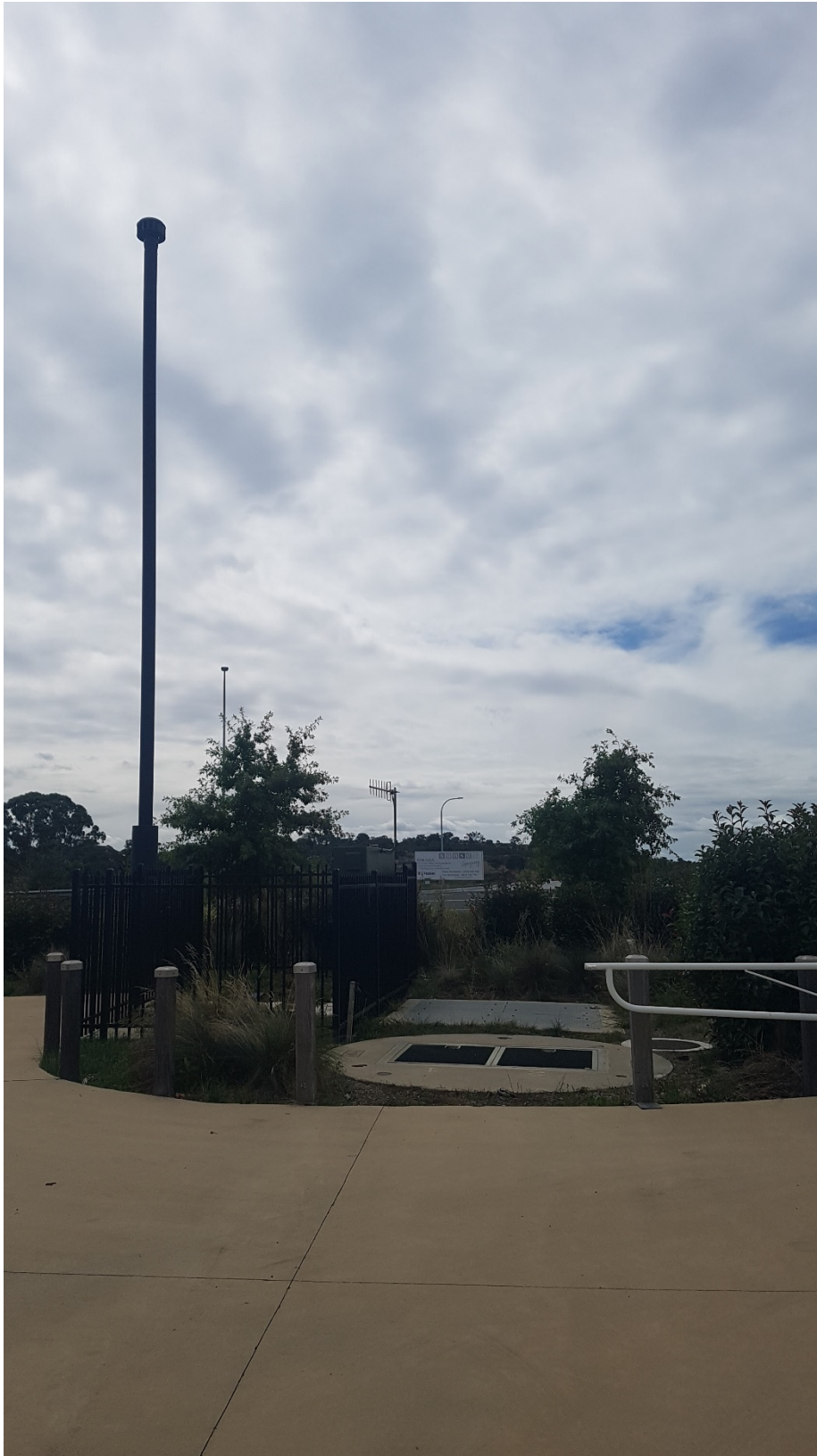
Figure 15-7 Googong SPS#1 elevated vent stack
