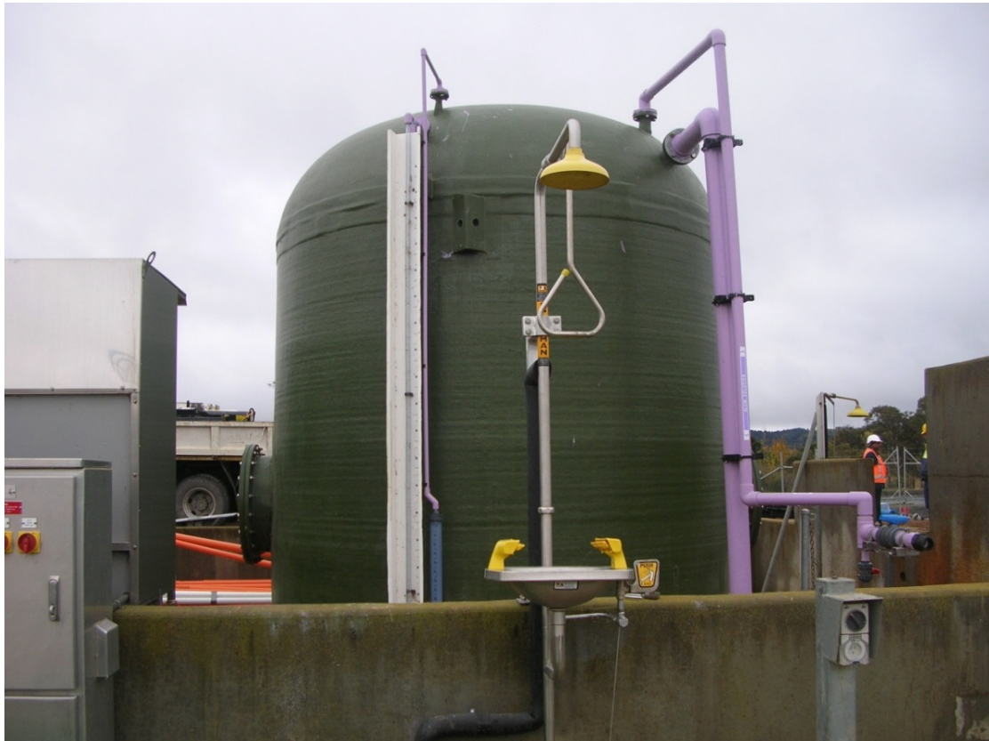
Figure 13 - 8: Bungendore STP – Chemical Storage Aluminium Sulphate
