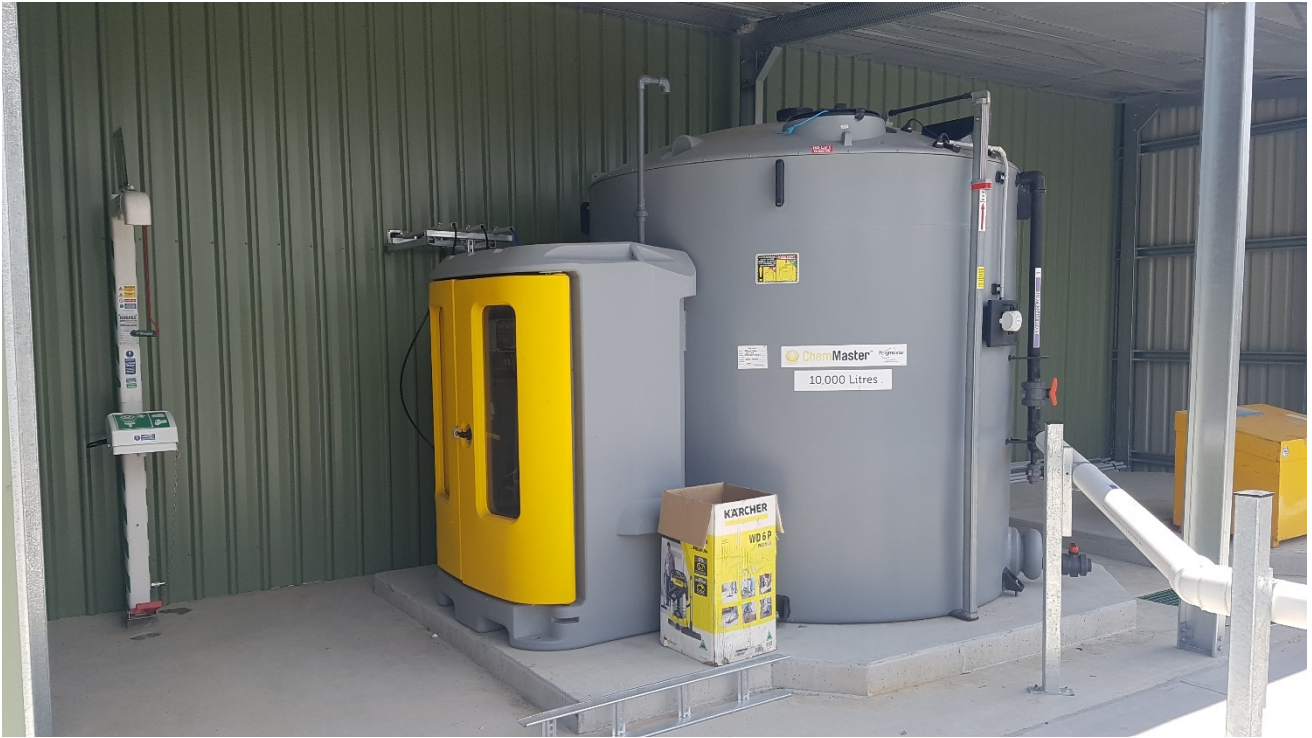
Bungendore recycled water system sodium hypochlorite storage tank
