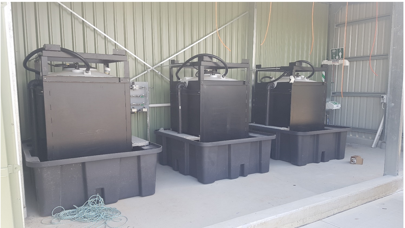
Bungendore recycled water system Citric Acid, NaOH and SMS storage tanks
