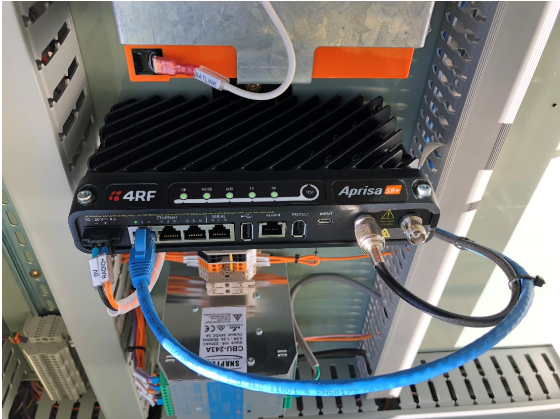
Figure 6 - 4: Telemetry Remote Terminal Unit (RTU)
