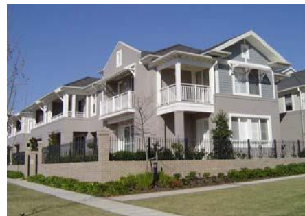
Façade treatment to address both streets. Articulated roof. Fences and landscaping defining the front boundary
