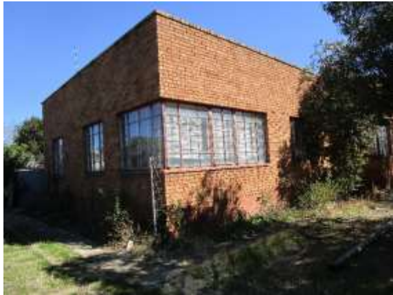
Crawford Street frontage and south side of cottage, showing square / rectangular massing, light-hued brickwork, parapet concealing roof and metal-framed windows
