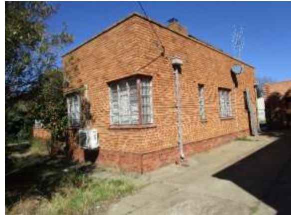
Crawford Street frontage and north side of cottage, showing square / rectangular massing, light-hued brickwork, parapet concealing roof and metal-framed windows
